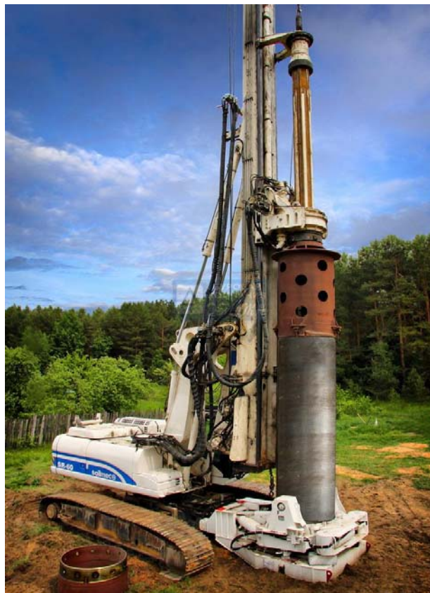
Figure 2, Installation using the Oscillator/Rotator Technique
