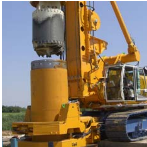
Figure 1, Drilling and Casing Installation using the Oscillator/Rotator Technique (Excavation Bucket Shown)
