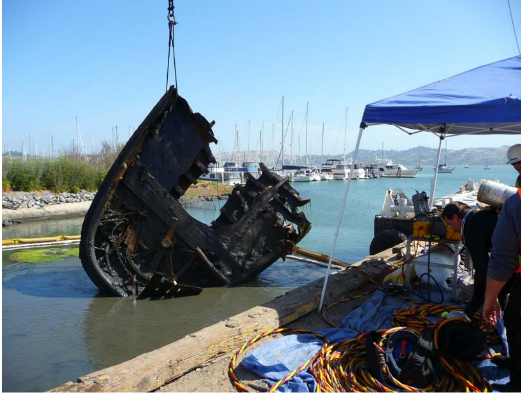
19. Last piece of the Tug Respect being removed by crane
