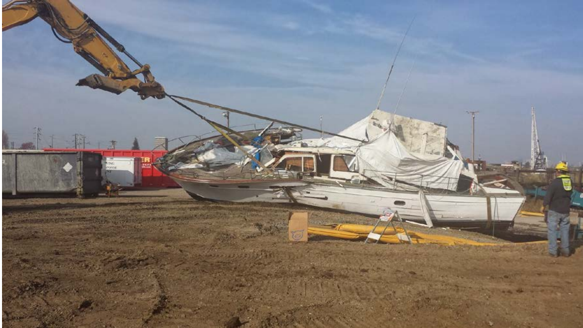
7. Vessel removal at Staging Area. Note: Vessel was not structurally sound to remove by boat lift.
