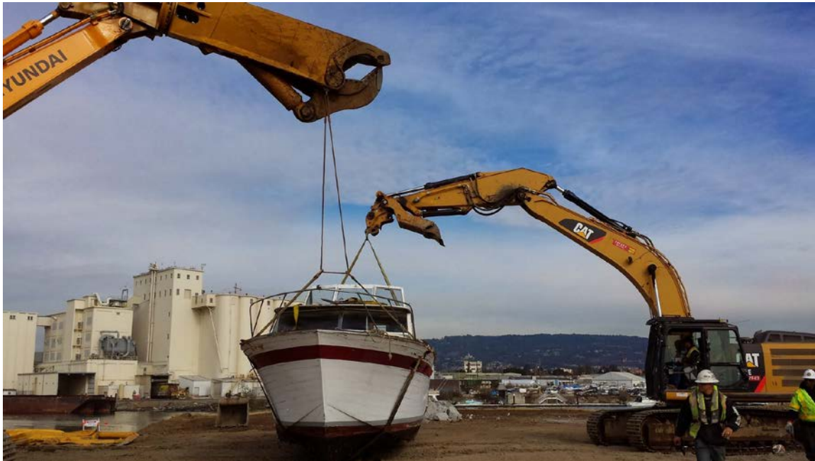
6. Vessel removal using two excavators at the Staging Area
