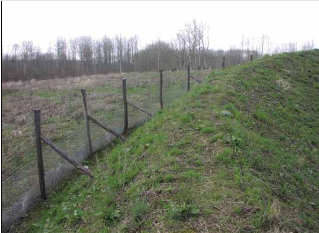
Figure 34. Photo. Berm on wildlife overpass (Credit: Tony Clevenger).
