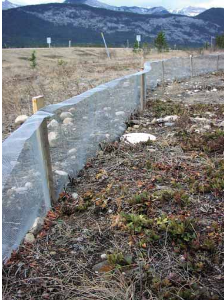
Figure 60. Photo. Barrier or drift fence for amphibians and reptiles (Credit: Tony Clevenger).
