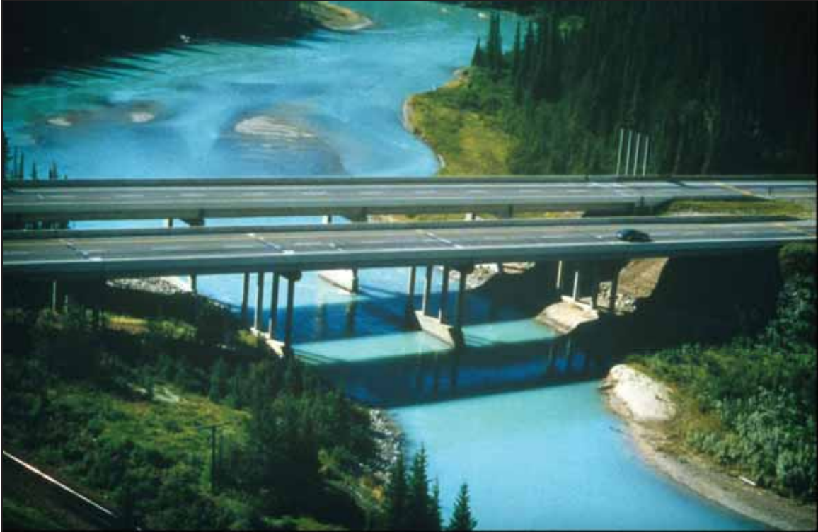
Figure 40. Photo. Wide span viaduct designed to conserve floodplain (Credit: Tony Clevenger).
