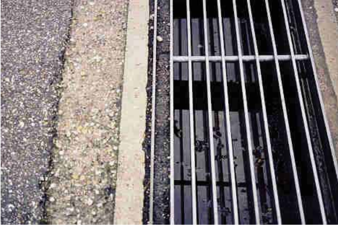
Figure 57. Photo. Grated slots on amphibian tunnels allows light and conservers ambient temperatures and humidity (Credit: Anonymous).
