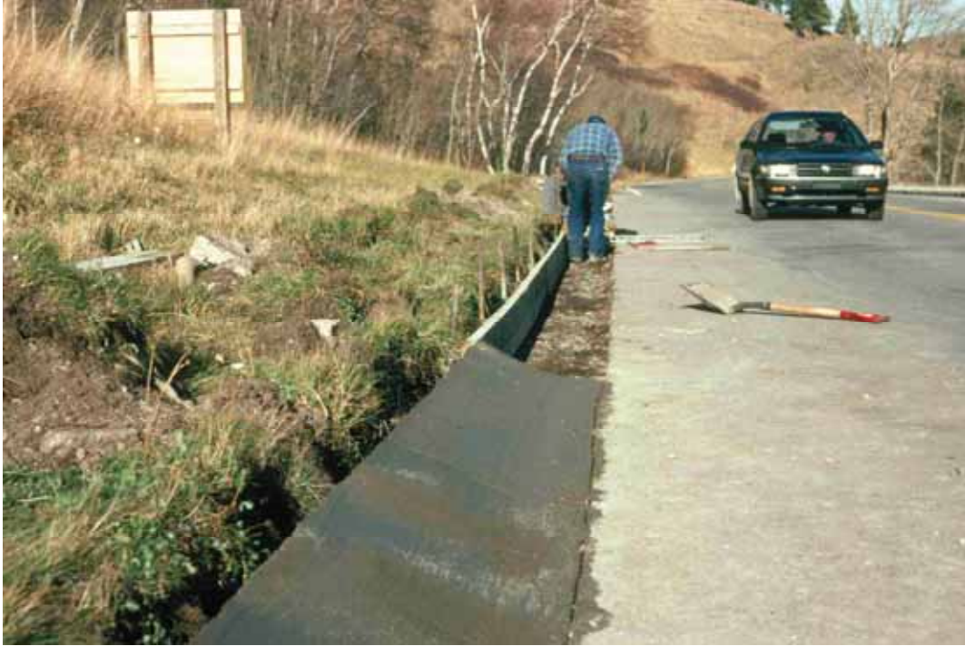
Figure 59. Photo. Construction of amphibian ramp to replace curb and allow cross-road movement of long-toed salamanders (Credit: Parks Canada).
