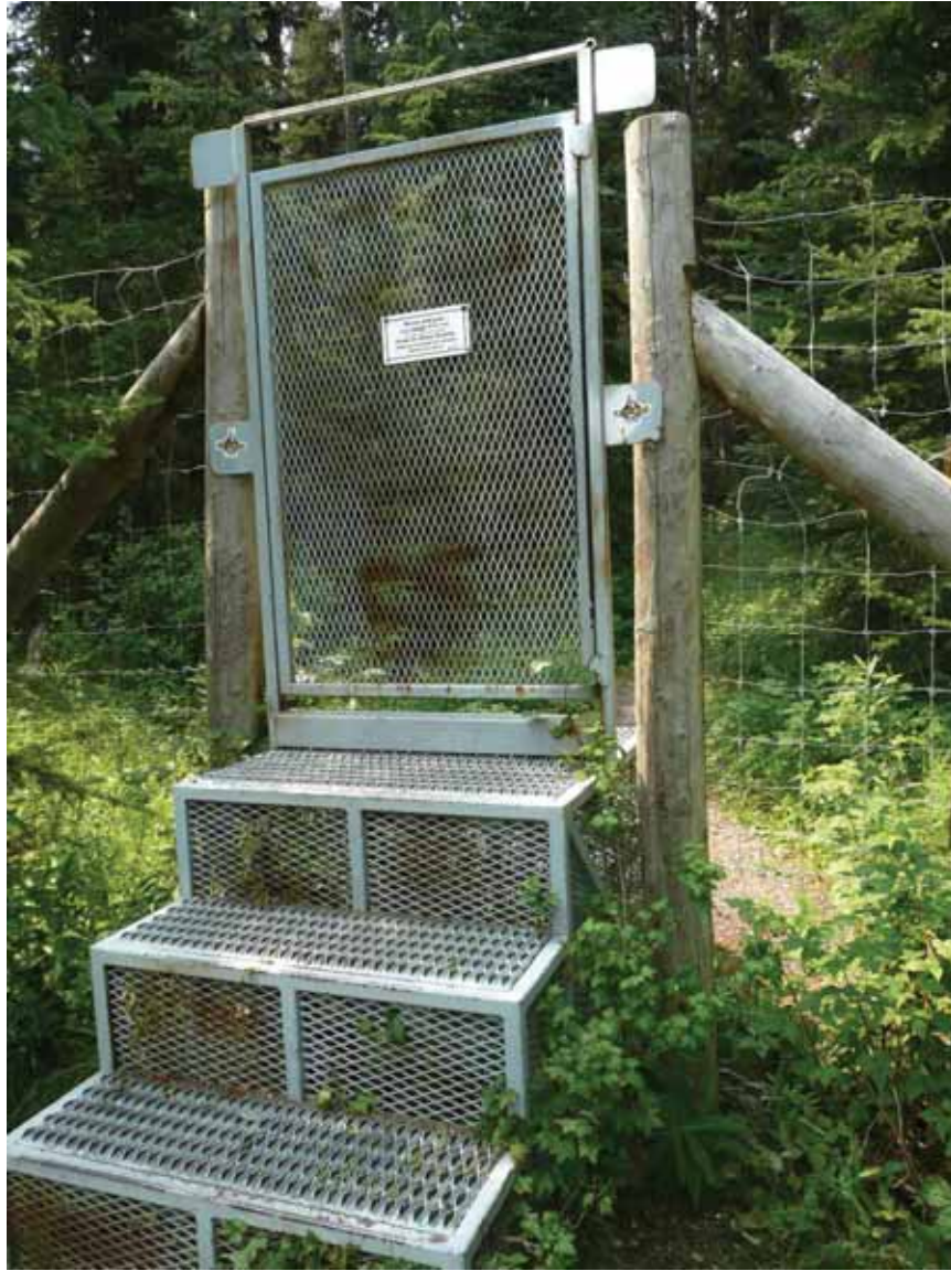
Figure 64. Photo. Step gate with spring-loaded door situated at trailhead in Banff National Park, Alberta (Credit: Tony Clevenger).
