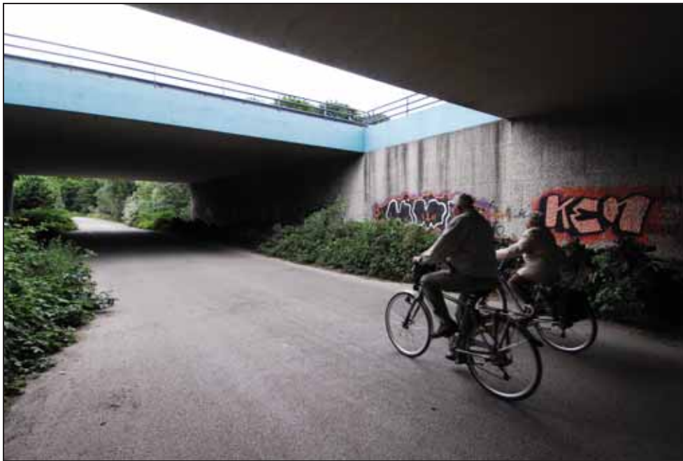
Figure 45. Photo. Multi-use underpass in The Netherlands retrofitted for human use and wildlife passage (Credit: Marcel Huijser).
