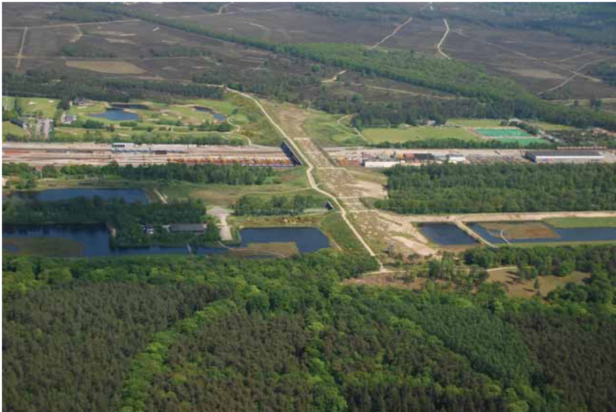
Figure 27. Photo. Most wildlife overpasses or landscape bridges are less than 70-80 m long; however, the one shown above near Hilversum, The Netherlands, is 800 m long and spans two roads and a railroad. (Credit: Goois Natuurreservaat, The Netherlands/Photo: W. Metz).
