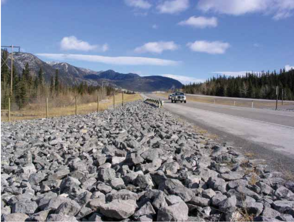
Figure 69. Photo. Boulder field at end of wildlife fence (Credit: Tony Clevenger).
