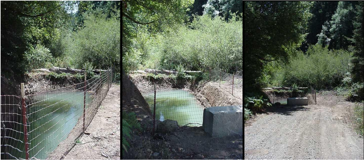
Sump by Mendocino Redwood Company near South Fork Albion River, August 2003
