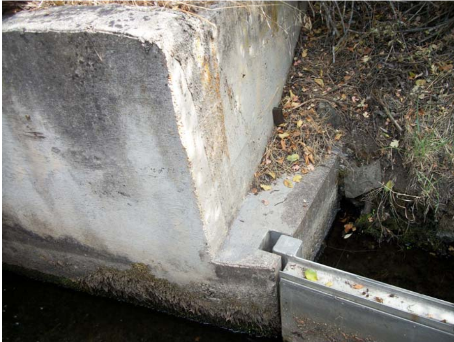
Site HR02. Roll Hart-01, Frame 13. Closeup showing concrete work and where the fish screen is anchored to it. View 104 degrees. 9/30/2016.
