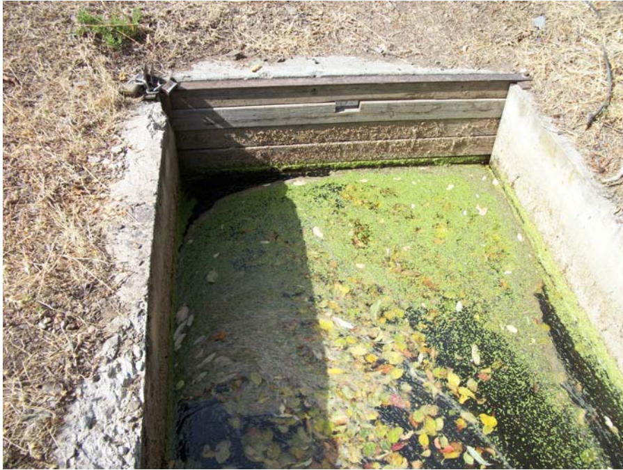
Site HR02. Roll Hart-01, Frame 15. View of overflow channel. Flows into a pipe just below the water surface. This pipe was likely the fish return pipe. View 318 degrees. 9/30/2016.
