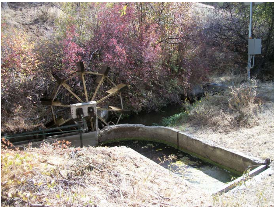
Site HR02. Roll Hart-01, Frame 07. Overview of south end of diversion structure. Diversion ditch is to right of water wheel. Flow meter and solar panel is at far right. View 160 degrees.
