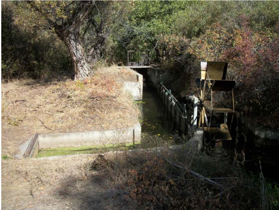
Site HR02. Roll Hart-01, Frame 06. Overview. Shows diversion structure with concrete retaining walls, undershot water wheel (allows for mechanical cleaning of fish screen), fish screen, and headgate. View 64 degrees.
