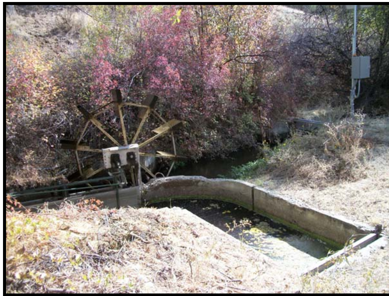
View of undershot water wheel with attached fish screen cleaning mechanism, overflow area leading to fish return pipe, and the modern gauging station.
