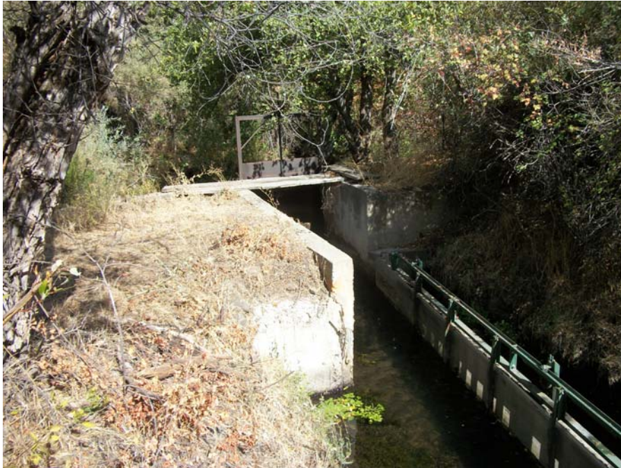
Site HR02. Roll Hart-01, Frame 08. View of diversion structure with fish screen on right and headgate in background, middle. View 170 degrees. 9/30/2016.
