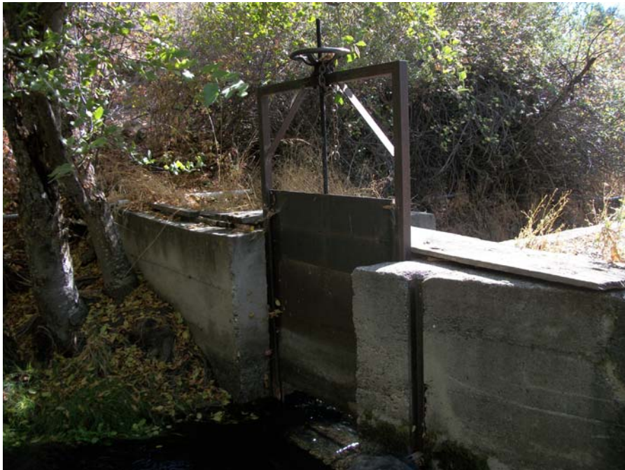
Site HR02. Roll Hart-01, Frame 09. North end of diversion structure showing concrete work, headgate, and wheel. Milled lumber forms were used when this part of the structure was built. View 164 degrees. 9/30/2016.
