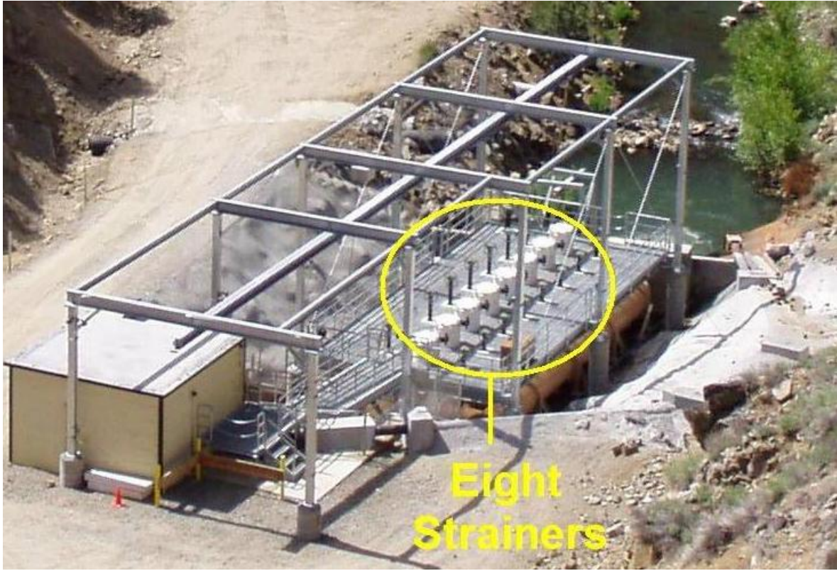
Figure 3 - Containment structure below Grizzly Dam at Lake Davis, California (DWR).
