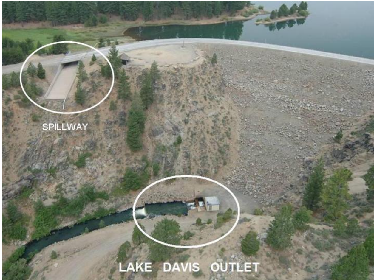
Figure 1 - Lake Davis showing Grizzly Valley Dam, the spillway, and outlet structure (pre-fish containment structure).
