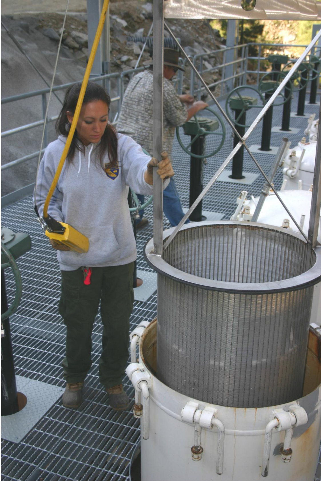
Figure 6 - Using mechanical hoist to remove strainer basket from containment structure.
