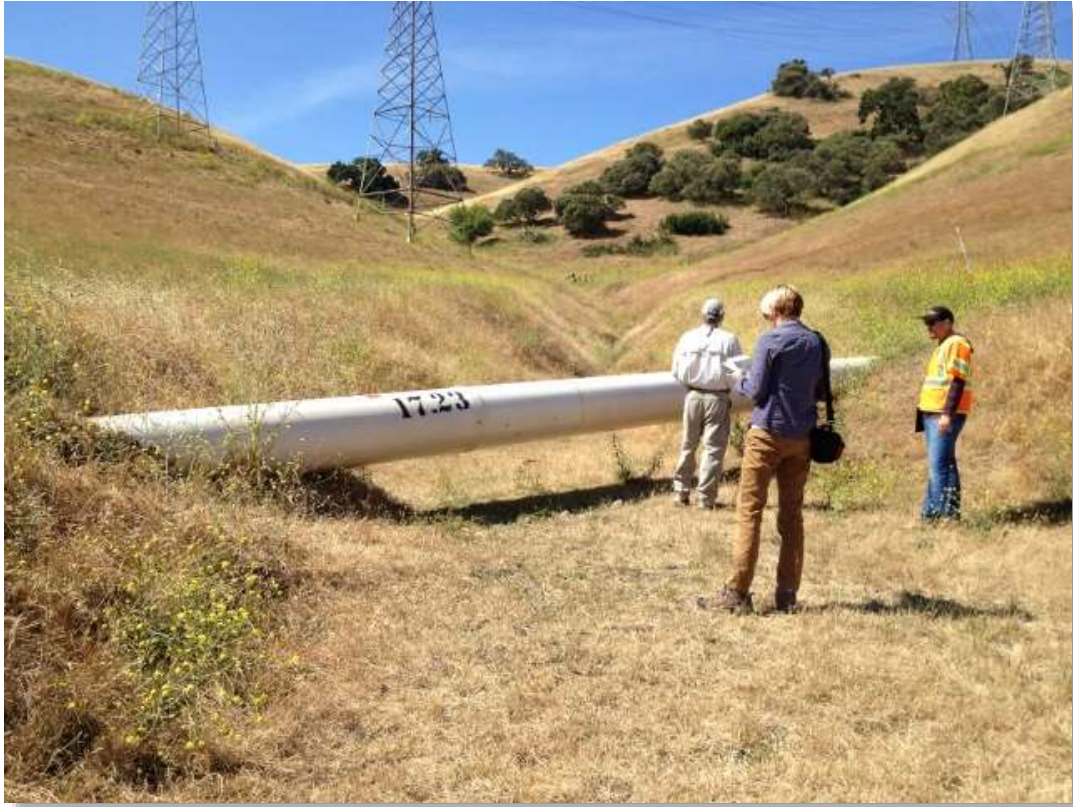
Work Areas 21-22, SAA Crossing, view southwest
