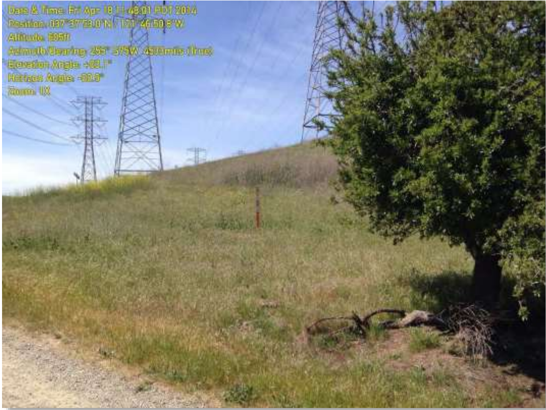
Work Area 18, view west
