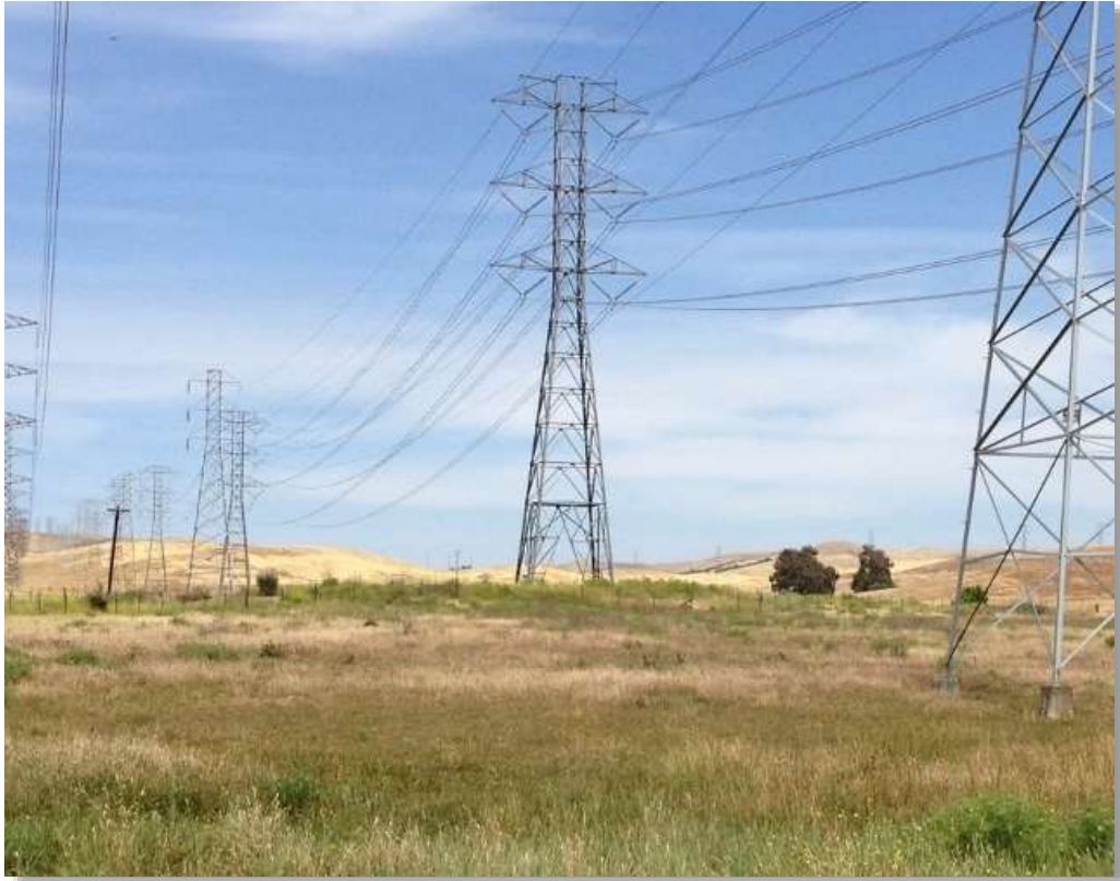
Work Area 36, view east-northeast
