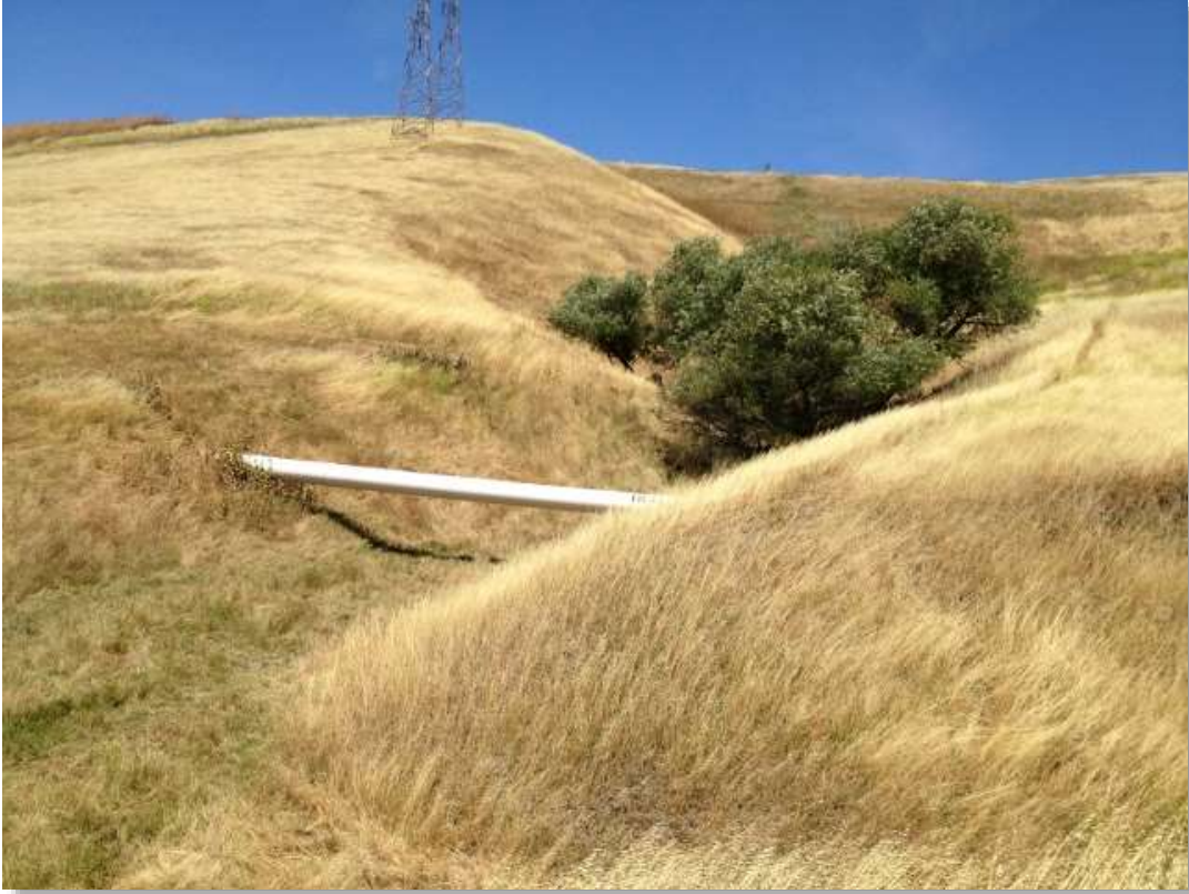
Work Area 24, SAA Crossing, view northwest
