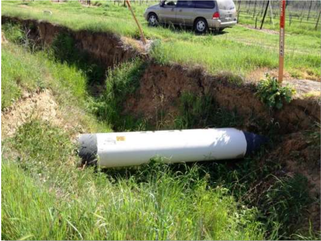
Work Areas 14-15, SAA Crossing, view southeast
