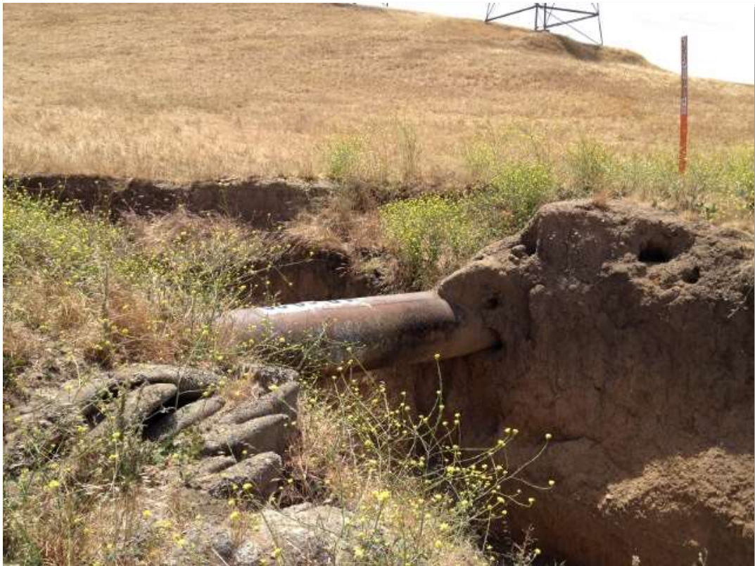
Work Areas 31-32, SAA Crossing, view south
