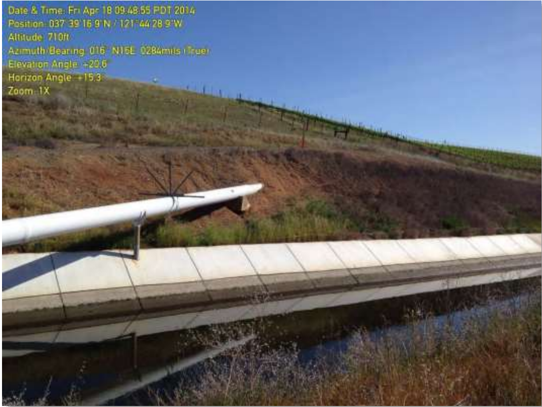
Work Areas 04-5, view north
