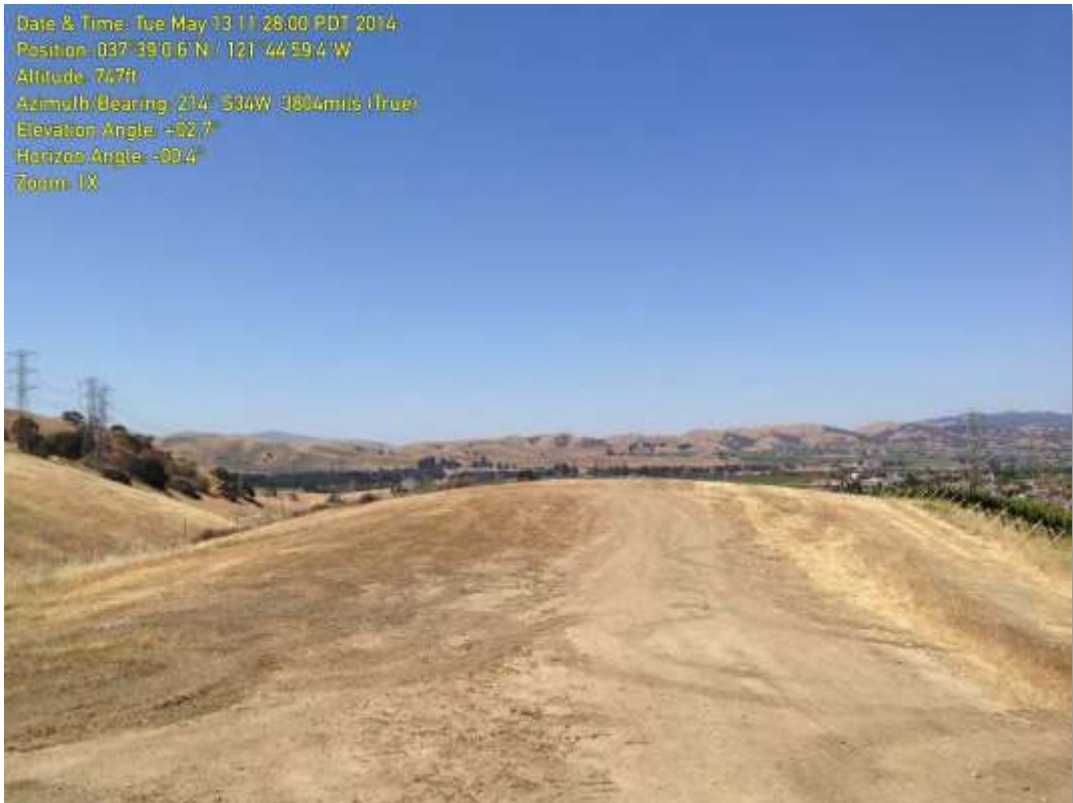
Work Area 08, view southwest
