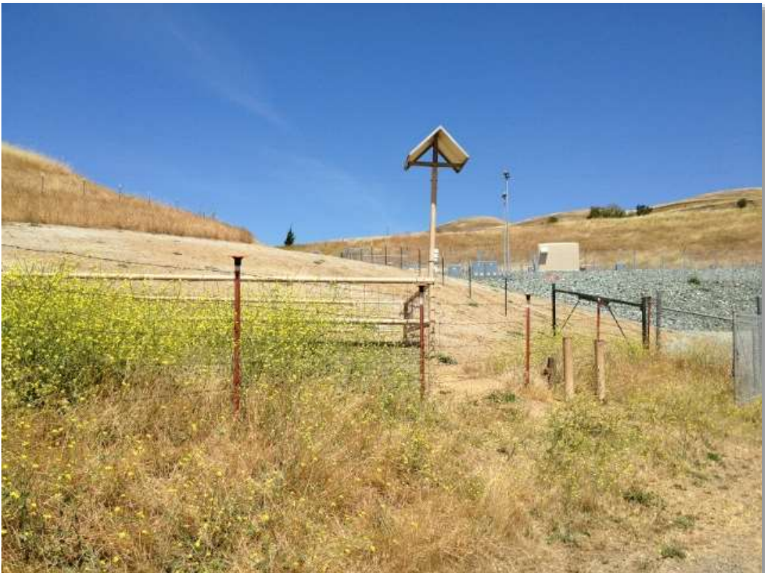
Work Areas 29-29A, view west-northwest
