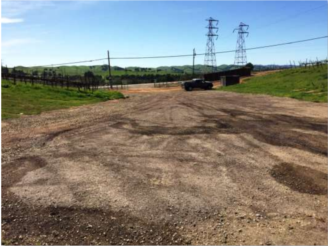
Work Area 12, view west-southwest
