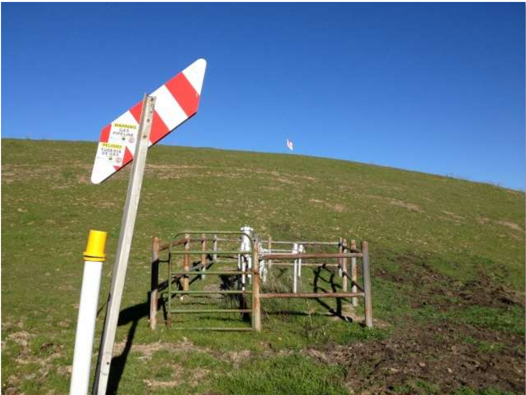
Work Area 62, Sheridan Valve Replacement, view east
