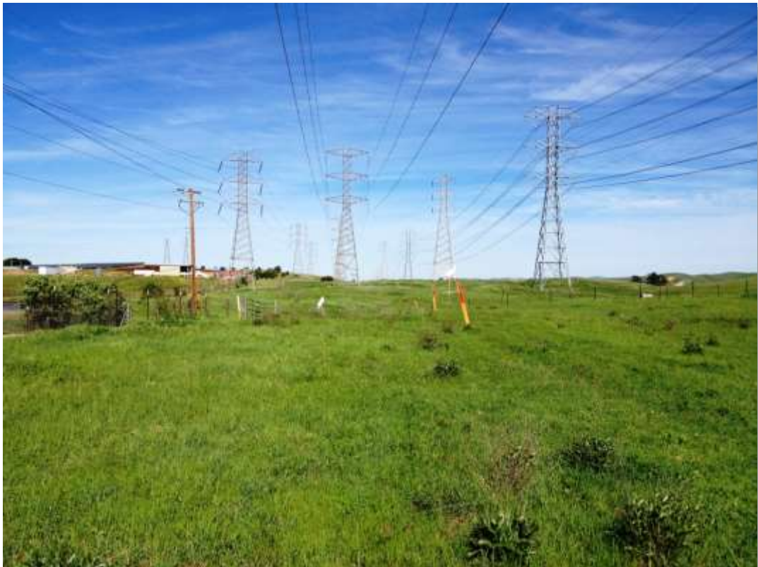
Work Area 19, view northeast
