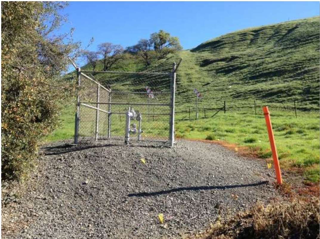
Work Area 41, view northeast-east
