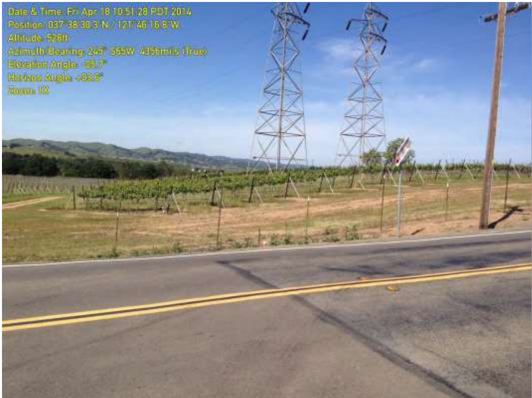
Work Area 13, view southwest
