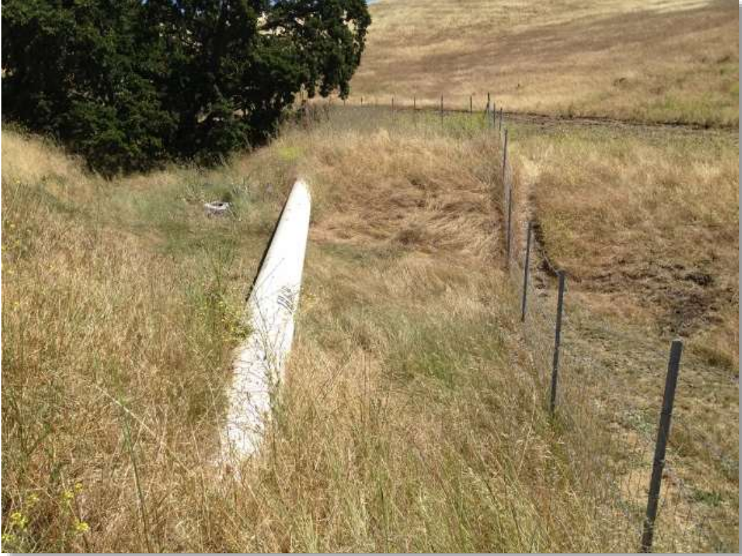
Work Area 28, SAA Crossing, view north-northeast
