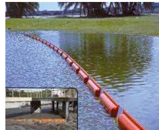
Fig. 3 External Tension boom
