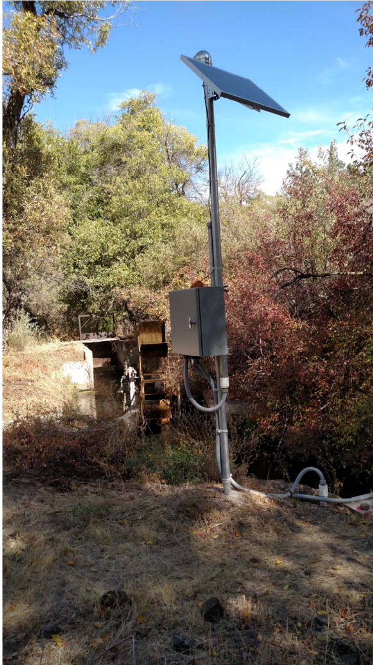
Site HR02. Roll Hart-01, Frame 17. View of flow solar panel with junction box. Connects to flow meter at surface on right. Site datum. 9/30/2016
