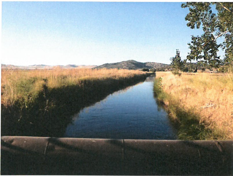
Photo 45 Facing north from south end of MWCD Wetland 2
