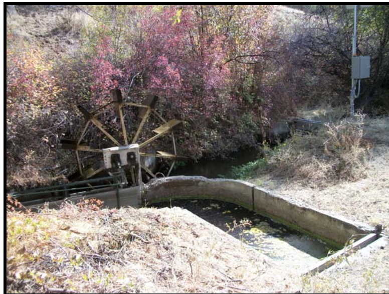
View of undershot water wheel with attached fish screen cleaning mechanism, overflow area leading to fish return pipe, and the modern gauging station.
