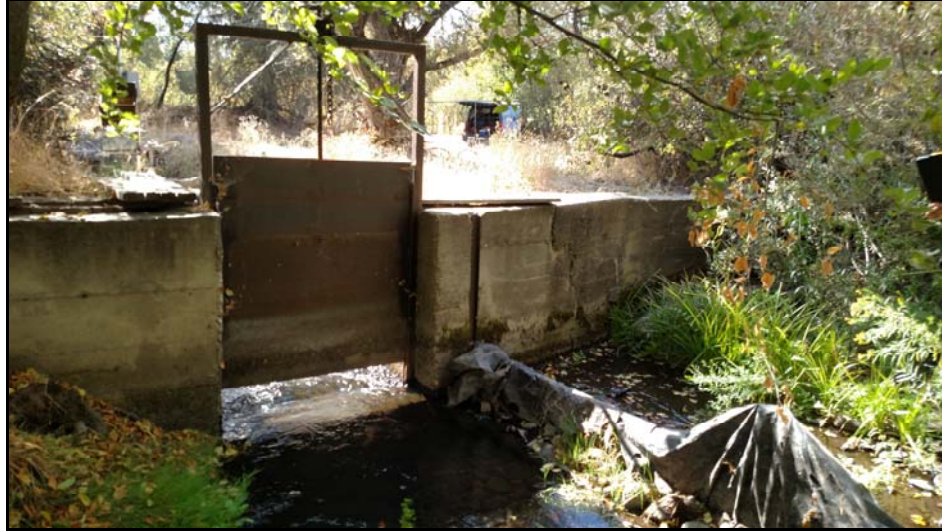
View of headgate, retaining wall, and plastic-covered plank check dam.
