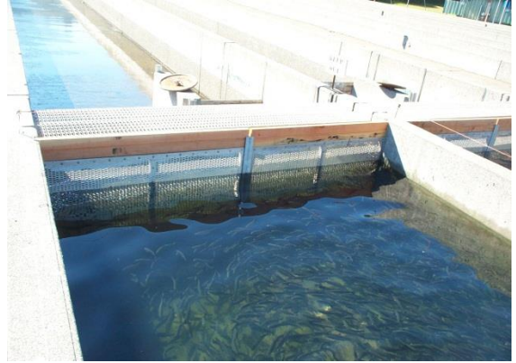
Figure 14. Raceway pond screen
