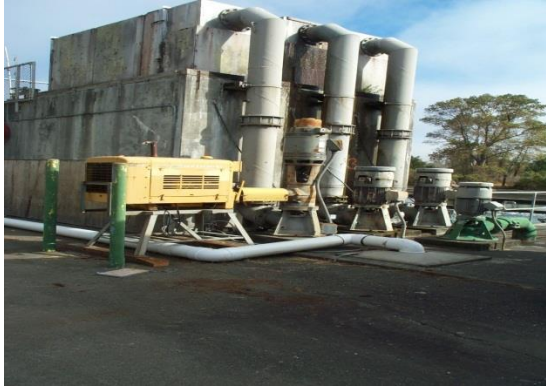
Figure 19. Primary pumps and sump
