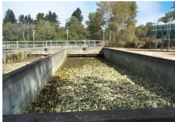
Figure 22. Oyster bed filtration system
