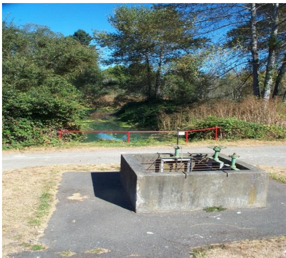
Figure 17. Settling pond head works
