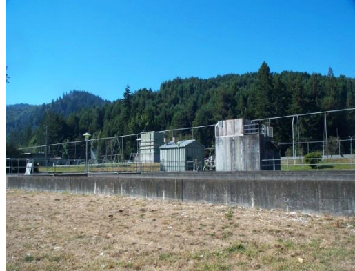
Figure 20. Secondary recirculation sump (right), pump house (center) and aeration tower (left)
