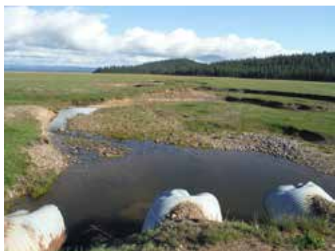
Figure 1. Looking down valley at the incised “Stroing Creek” channel from the road, within the Greenville Creek project area, showing the expansive floodplain and damaged road culverts.
