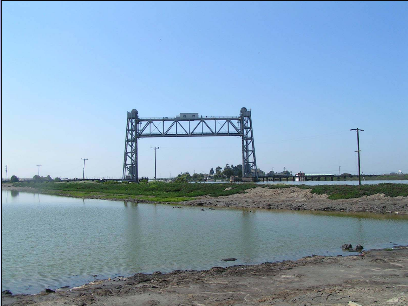
Northwestern corner of pond 9 (looking south)
