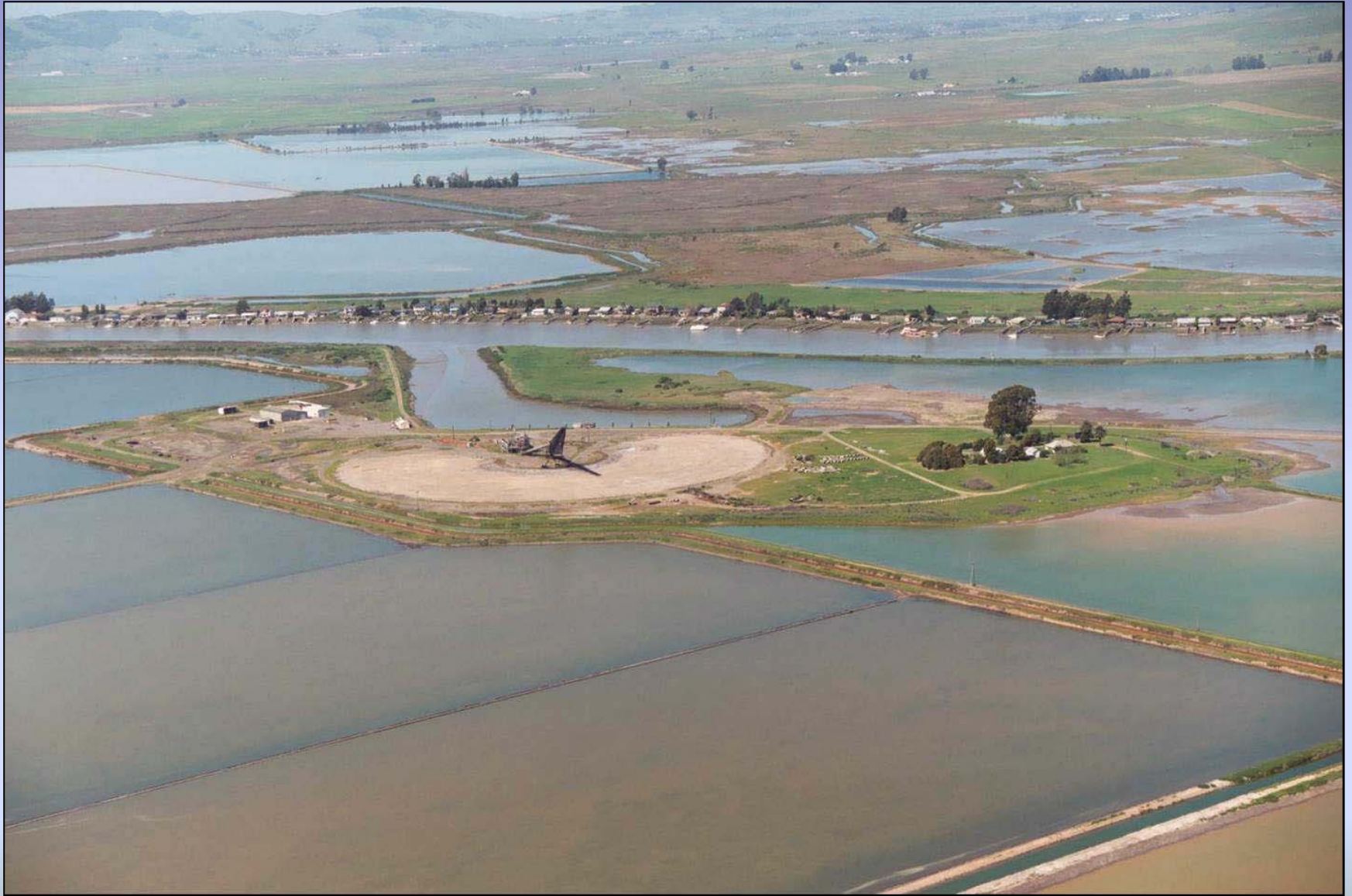
Overhead view of wash pond area of Phase 1 Restoration
