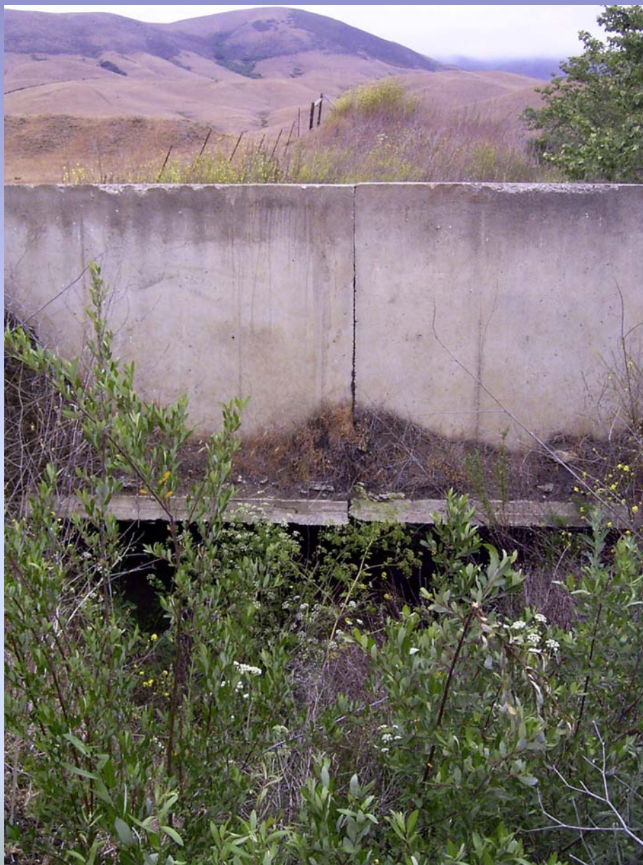
Concrete Headwall at Site 5
