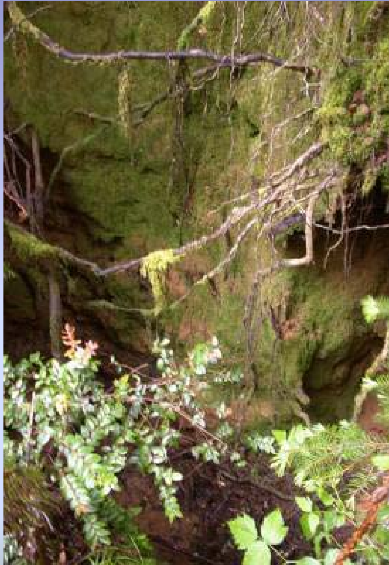
Green Creek #407: 12ft deep headcut in erosion ditch caused by diversion of stream channel.
