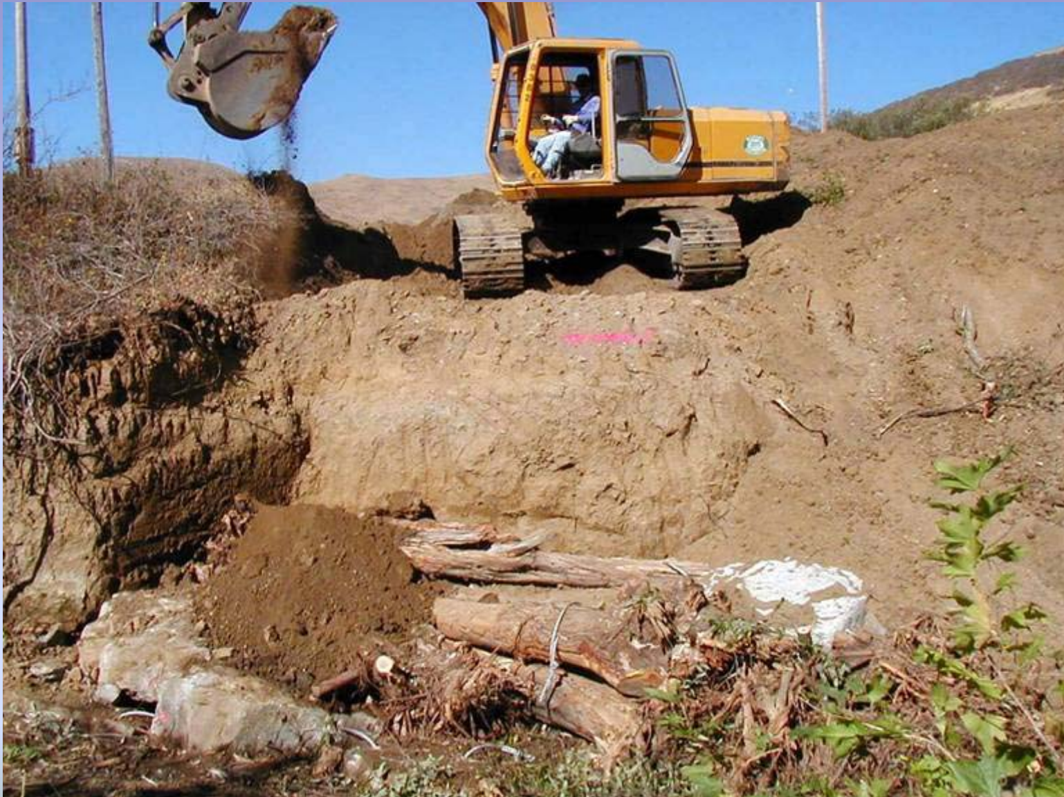
Eroded bank during repair work
