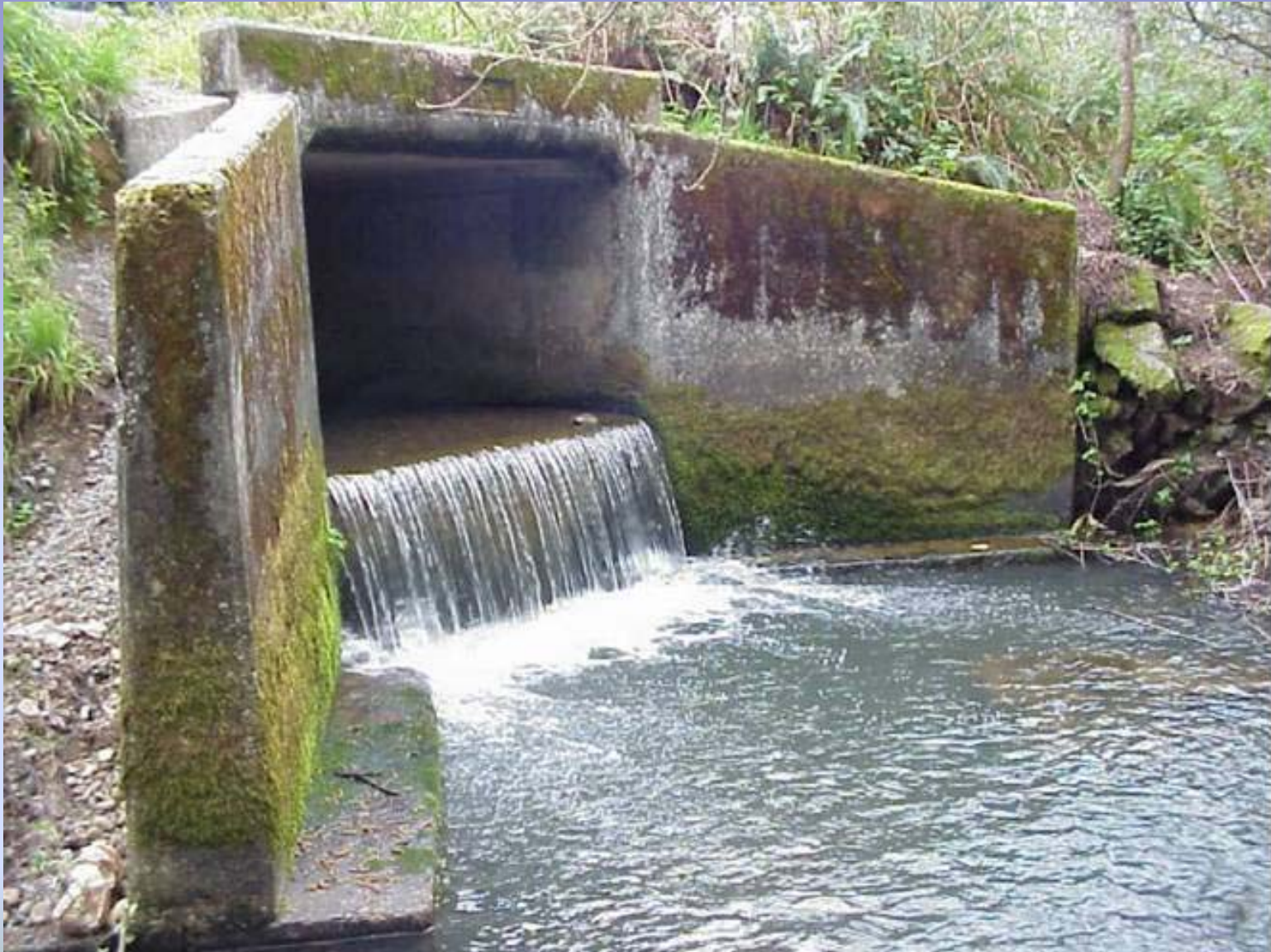
Culvert fish barrier prior to restoration
