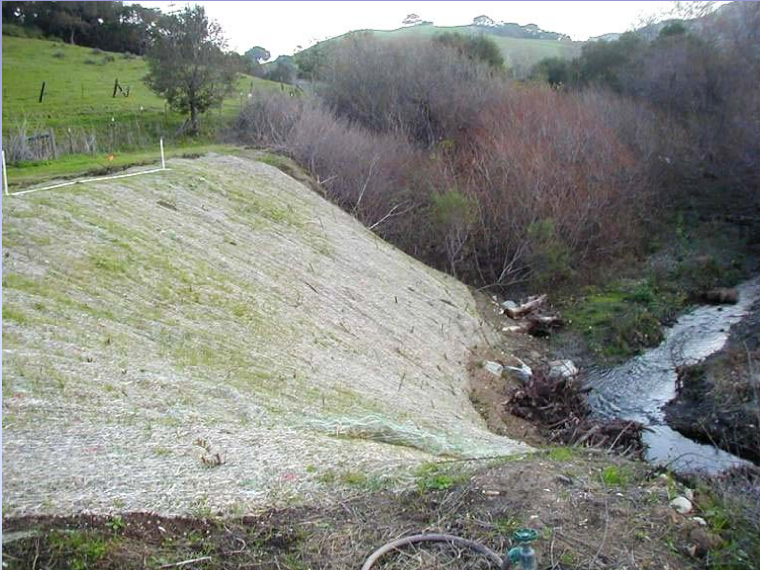
Eroded bank following repair work and seeding
