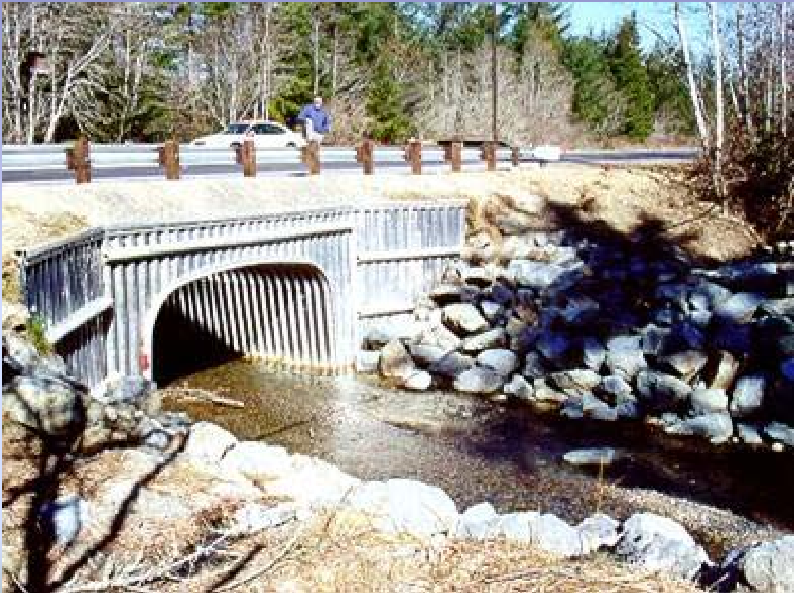
Culvert after repairs; now will allow fish passage
