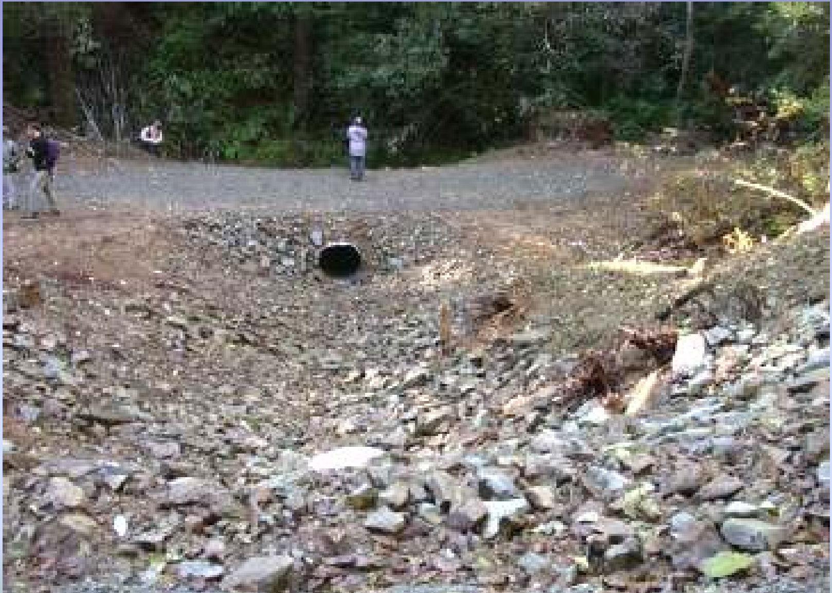
Green Creek #407 & 413: Completed sites with rock armoring around culverts and connecting stream channel.
