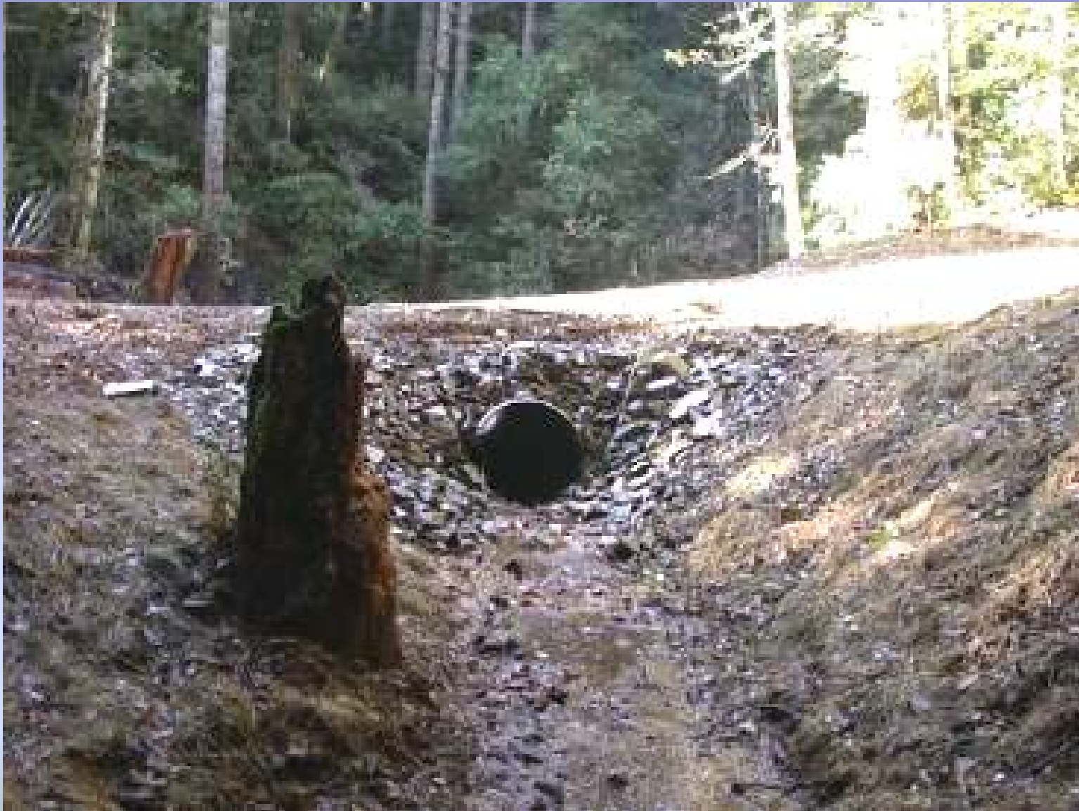
Green Creek #407: Completed site with rock armoring around culvert.
