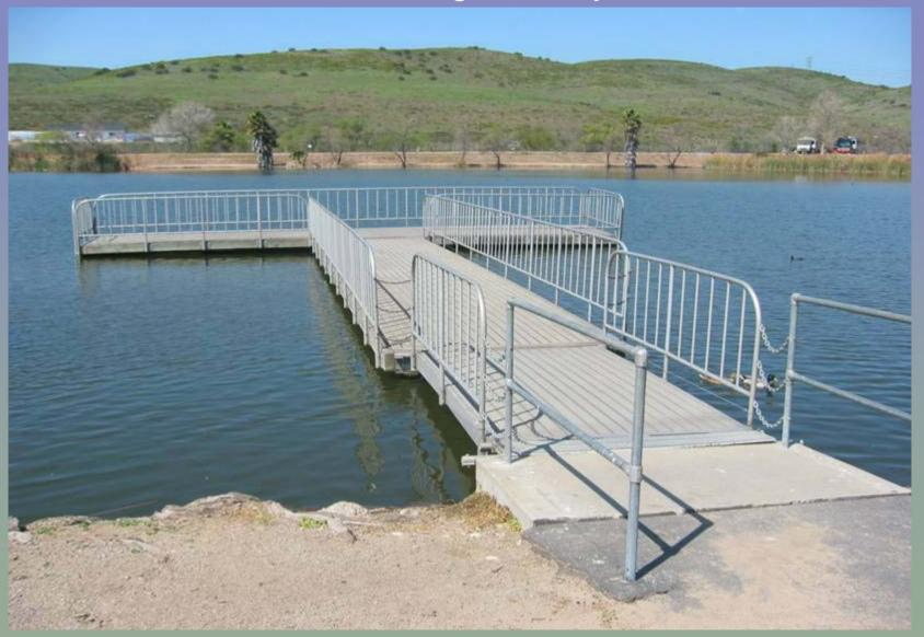
This is one of the two piers to be replaced; the vertical posts are supporting the end of the pier because the floats underneath have deteriorated.
