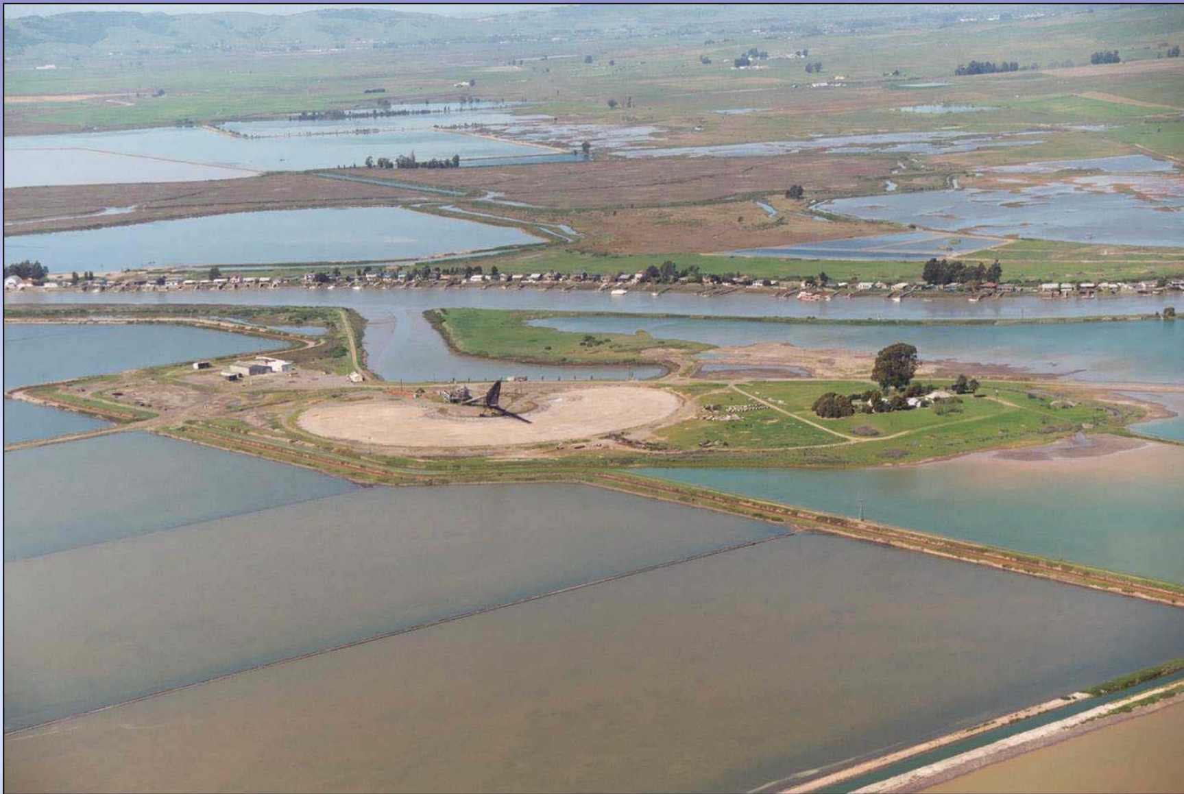
Aerial view of wash pond area of Phase 1 Restoration
