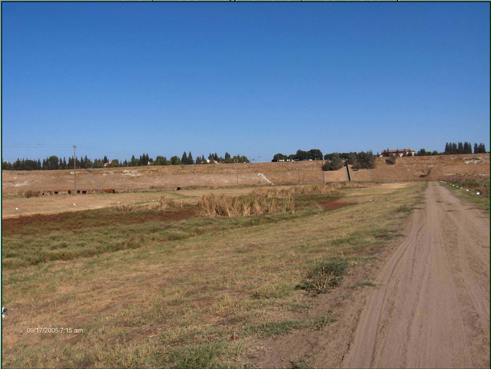
Stormwater treatment channel at Jensen River Ranch
