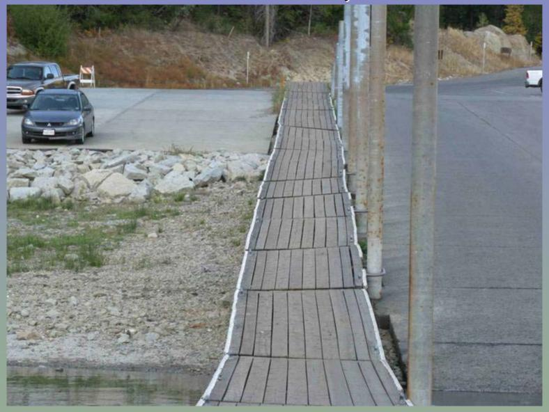
All the boarding floats are warped and in need of replacement.
