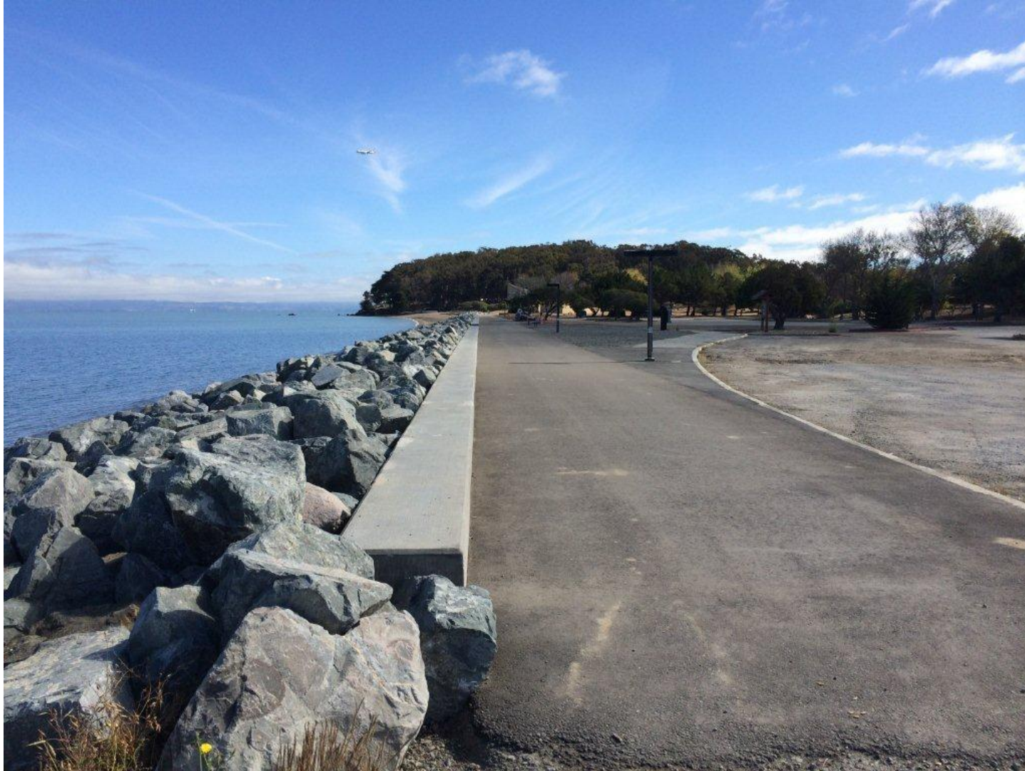
Image 8: View of Promenade showing newly paved trail that links to other park pathways (post project). Photo shows new curb/seating wall and adequate revetment.
