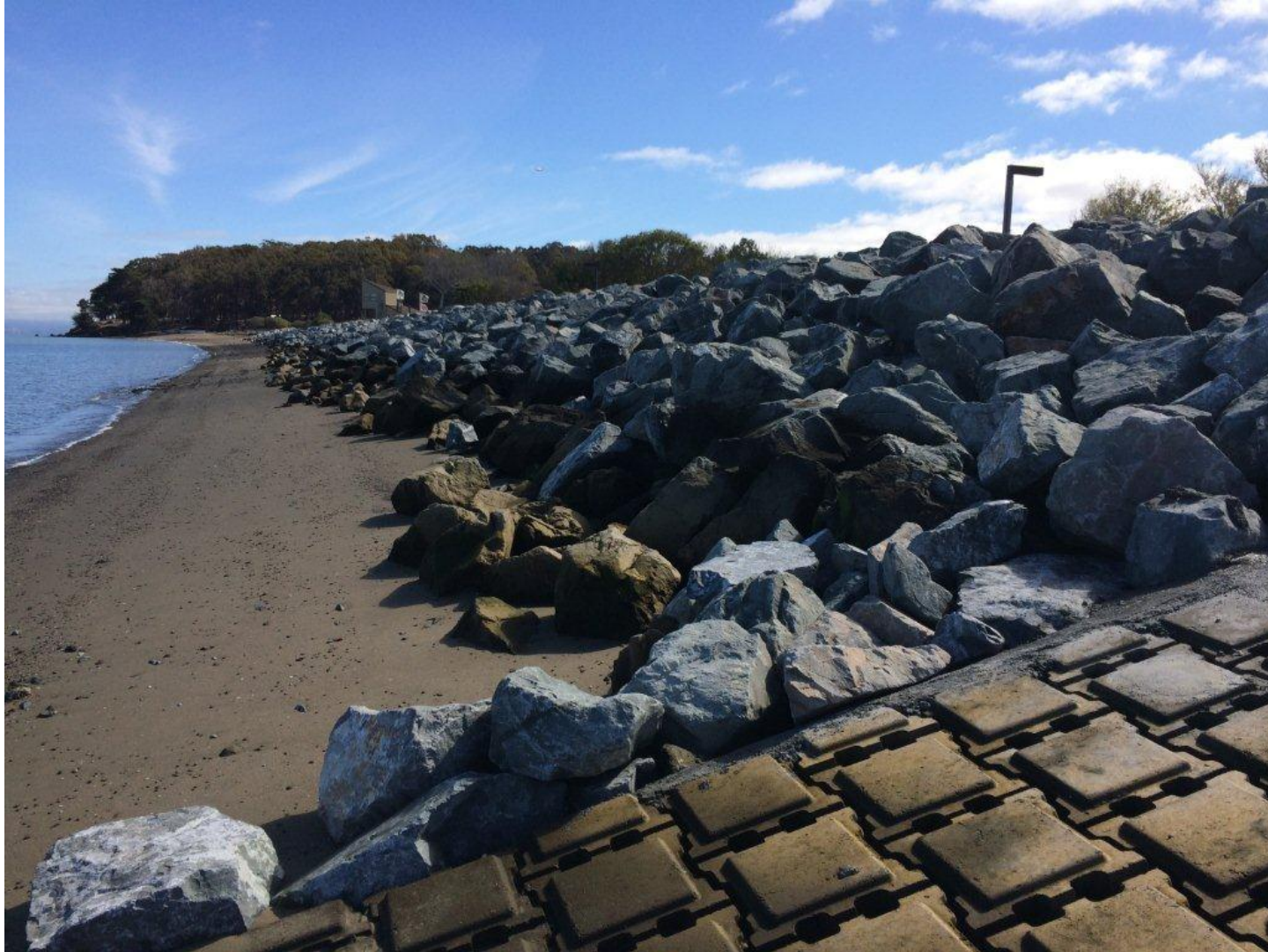
Image 7: View of another new ramp and shoreline revetment built to withstand tides and wind (post-project).
