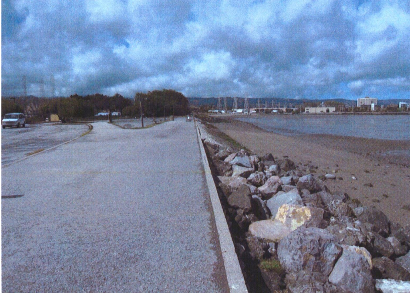
Image 3: Prior to the project, revetment boulders were no longer in effective placement to protect the Promenade. In addition, Promenade trail users had no curb between the trail and revetment.
