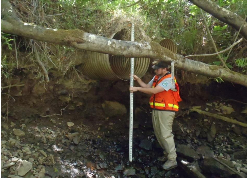
Photo 1: Outlet of culvert (Habitat Unit #3)
