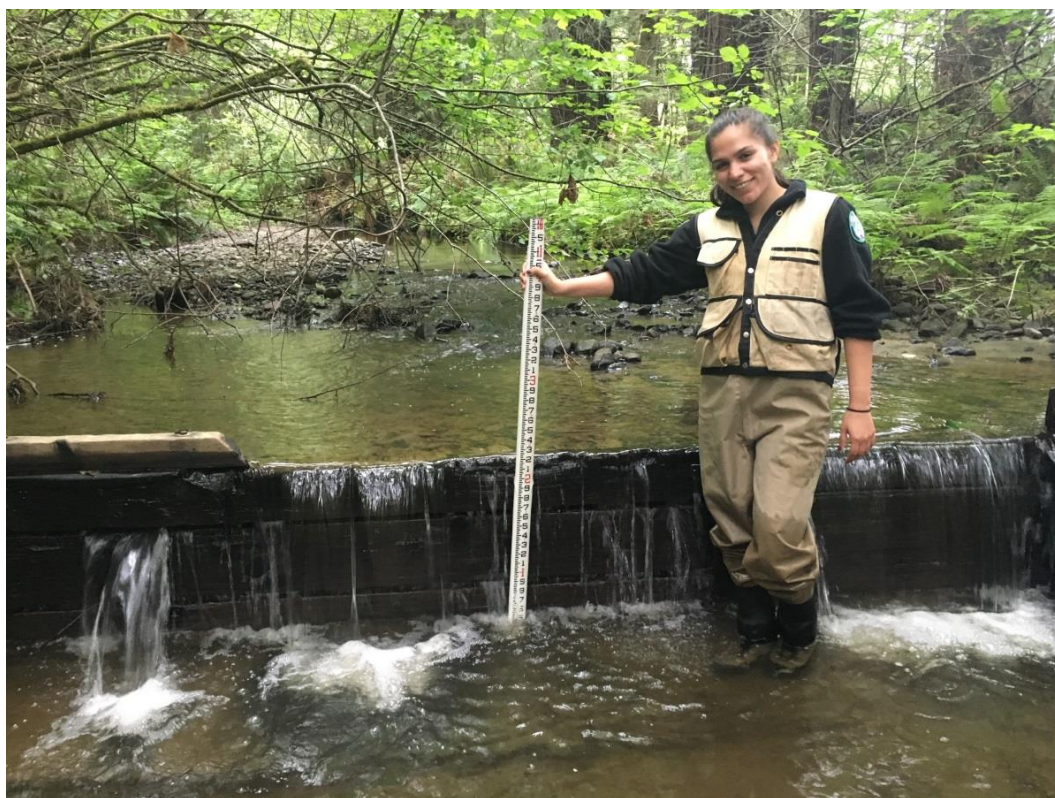
Photo 1. Wooden weir (Habitat # 0071.00) that forms seasonal barrier. Structure was formerly associated with the PALCO fish rearing facility that is no longer in use. Photo taken 5/25/2016.
