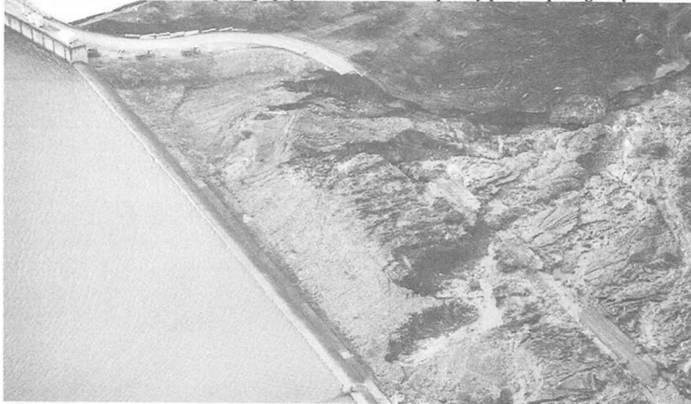
Major sinkhole on spillway at Lake Oroville
