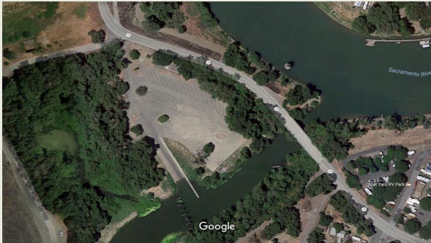
Aerial view of the project area
