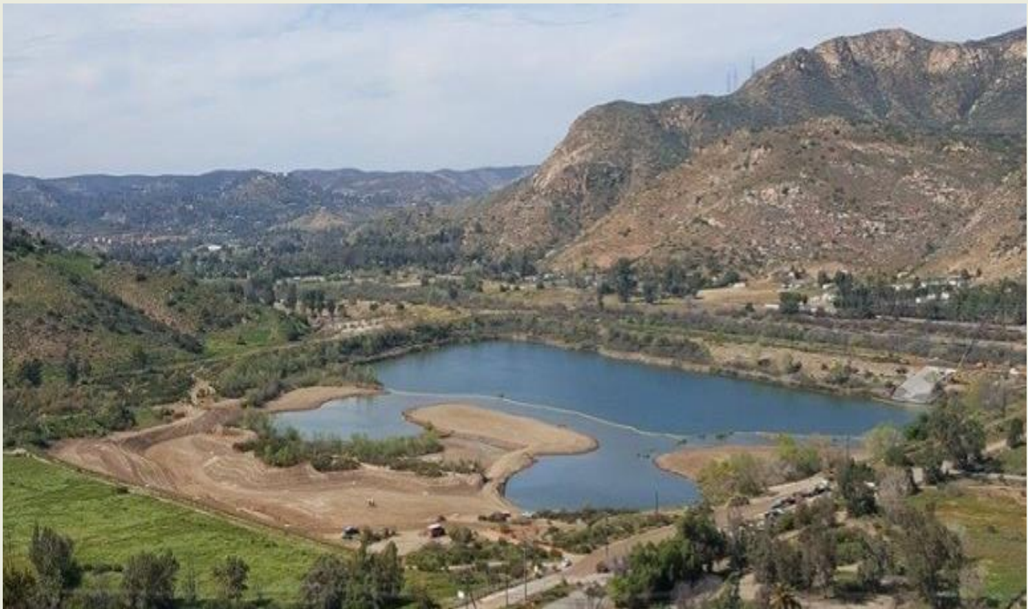
Project site: Post-Construction
