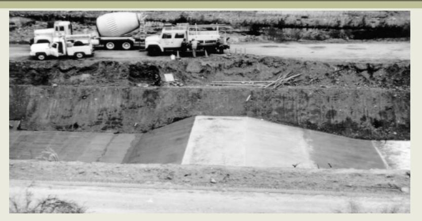
A broad crested weir (BCW) being built. BCW's will be installed to increase the accuracy of measuring how much water 3 state wildlife areas are receiving.
