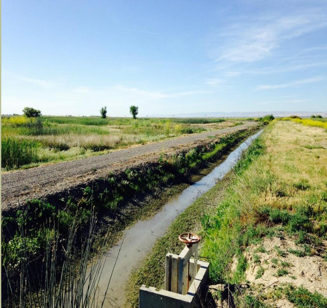
A section of the main delivery ditch bank on the Gadwall Unit will be built up to allow the wildlife area staff to build up head pressure to push water into adjacent units. Currently, water almost floods over the existing ditch bank (left side of picture) when building up head pressure.
