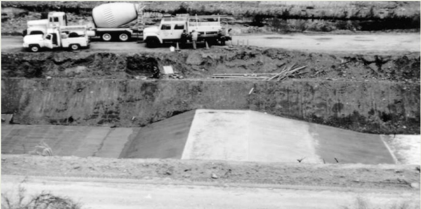
A broad crested weir (BCW) being built. BCW's will be installed to increase the accuracy of measuring how much water 3 state wildlife areas are receiving.
