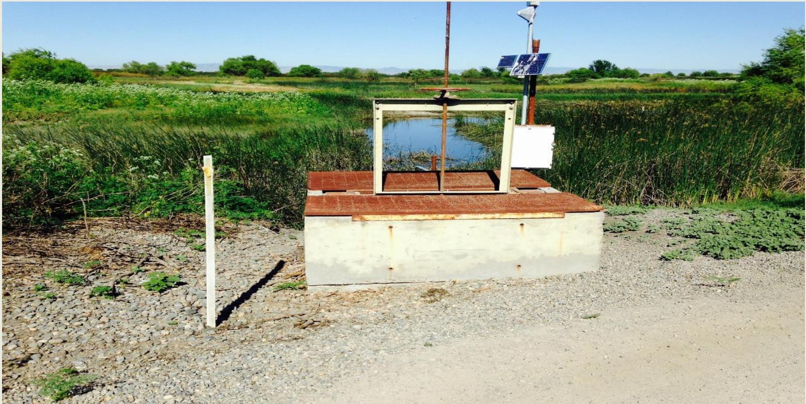
The current drainage structure at Buttonwillow Lakes Dam on Los Banos Wildlife Area. We will rebuild the dam to allow for a dropdown gate to be installed.
