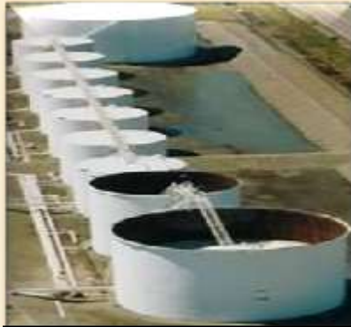
Tank Farm Monitoring
