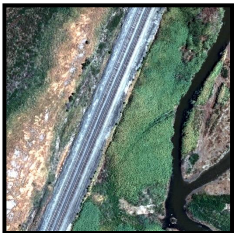
Railroad track, ballast and roadbed.
