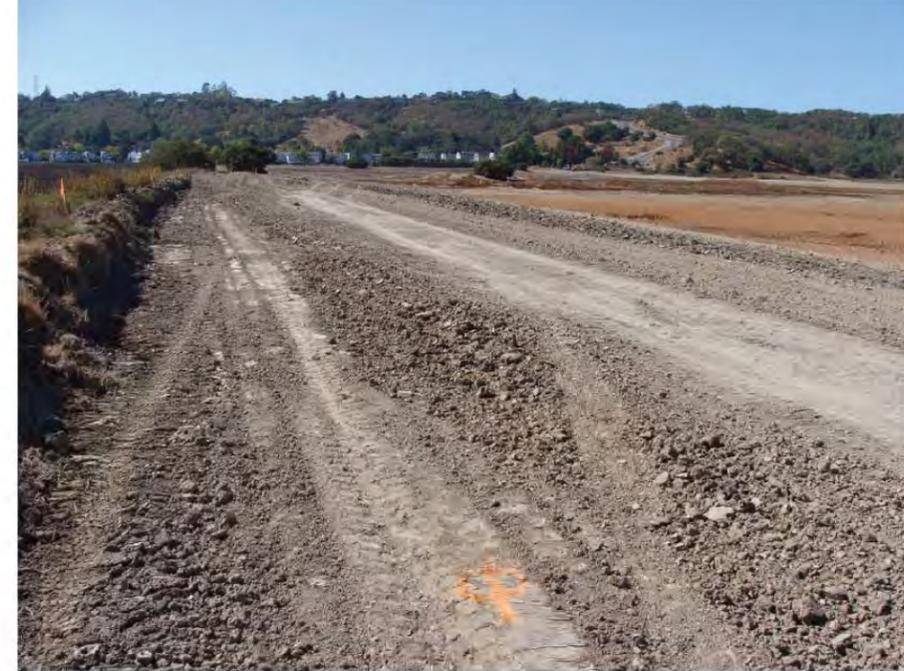
The photograph shows the same levee close to the end of Phase 2 construction, with the levee crest lowered to high tide except for a small "check berm" to prevent overtopping. Note: The tidal boundary is on the left, opposite of the drawing.
