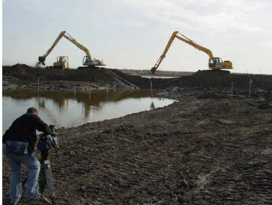
Two long-reach excavators and a low ground pressure dozer excavate a breach. Not seen is a third long reach excavator that re-handled the excavated material to spread it further, and additional dozers that helped spread the material. Ideally, the breach is constructed in a few hours, between high tides, including while water flows through. When multiple days or longer are required, flows through or over the breach are controlled to avoid failure of the breach.
