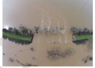
Figure 6: Levee failure at MWT during 2017 floods. Photo: J. Grossman - TNC
