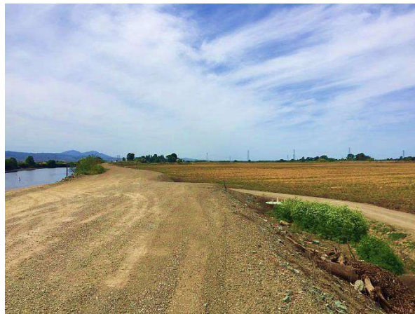
Figure 4: South Delta levee road
