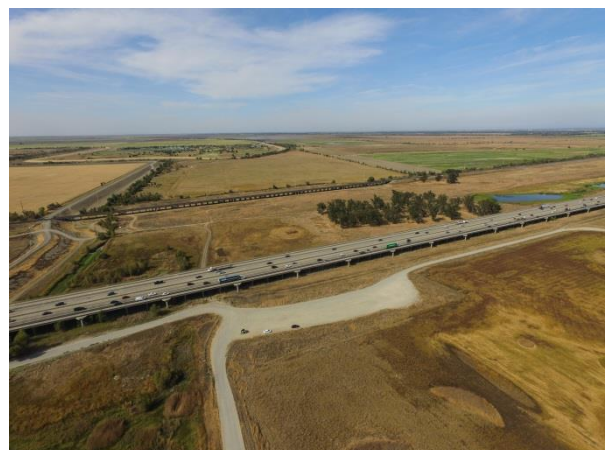
Figure 6: Highway 80 crossing Yolo Bypass looking north
