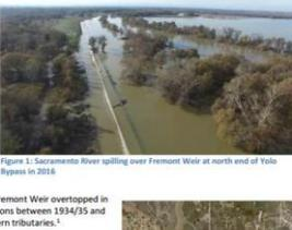
Figure 1: Sacramento River spilling over Fremont Weir at north end of Yolo Bypass in 2016.
