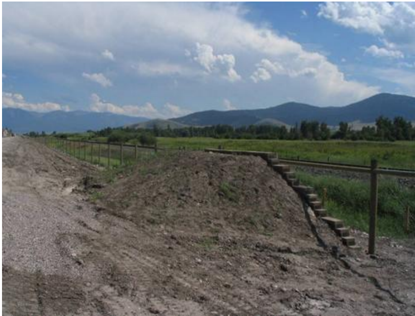
Figure 26. Dirt jump-outs on I-93, Arizona (Photo: http://www.fhwa.gov )
