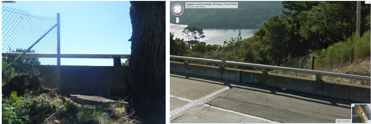
Figure 29. Fence-lines joining bridge abutments creating tie-in points for deer-proof fencing.
