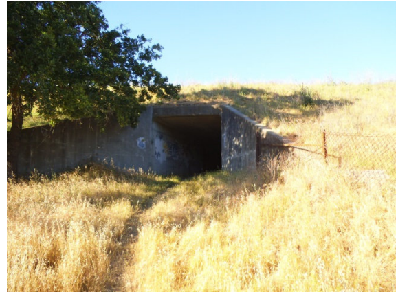
Figure 5A. Box culvert at Sandhill Road
