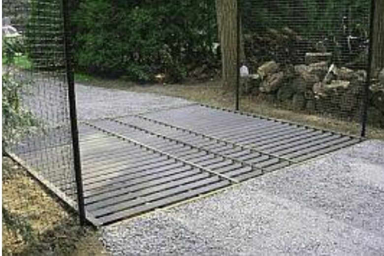
Figure 27. Cattle-guard linked to 8-foot fence to prevent deer from entering a road-way around the ends of a fence.
