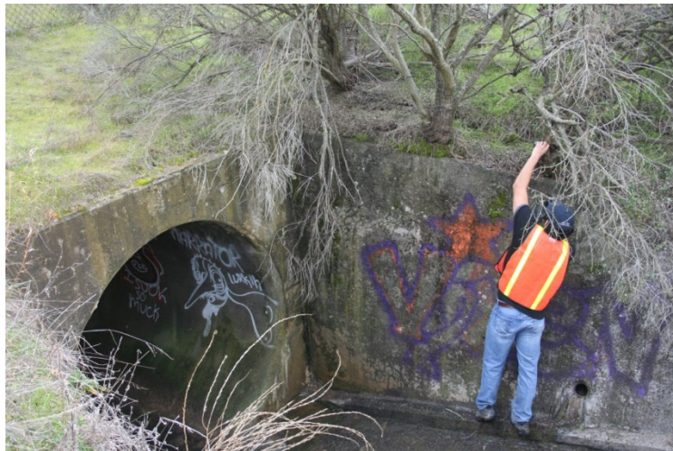
Figure 5B. Road Ecology Center staff at round culvert at Sandhill Road
