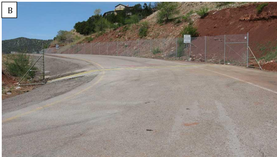
Figure 28. (A) Electrified mat deployed across an asphalt road. (B) Electrified mat associated with adjacent fences.
