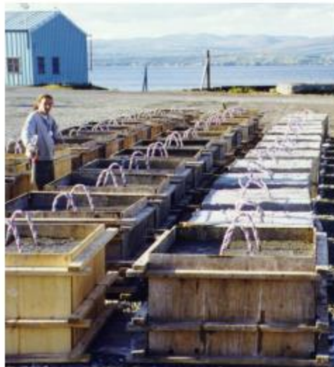
Figure 17. Plywood and lumber forms for the construction of concrete moorings
