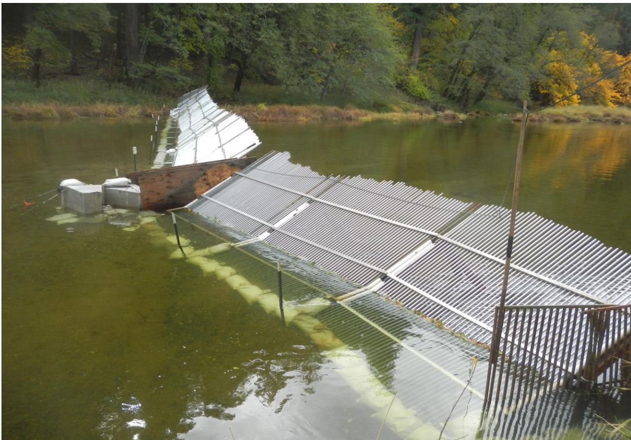
Figure 2. Scott River Fish Counting Facility located in Siskiyou County, California, 2016.
