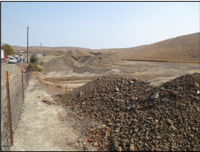
Photo 3. Occurrence 1: Greenville Road on September 24, 2014, view direction North-northeast
