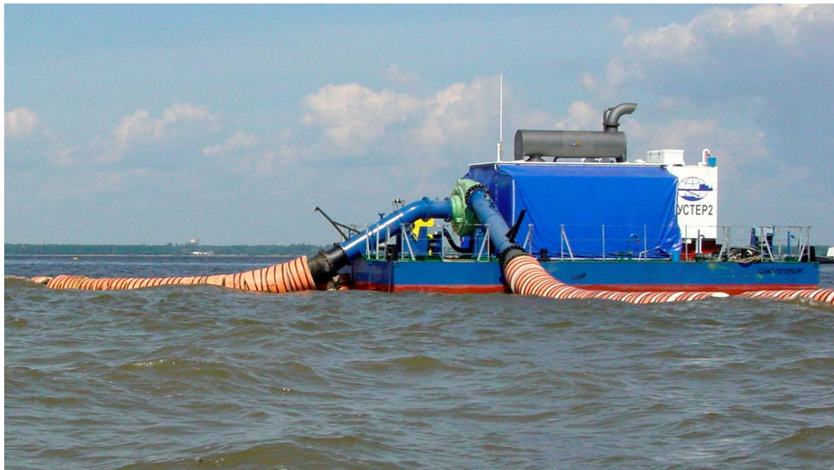
Figure 4-4: A typical booster station, used to improve sediment discharge production rate
