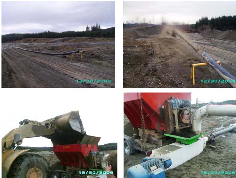
Figure 4-9: Pneumatic sediment conveying system
