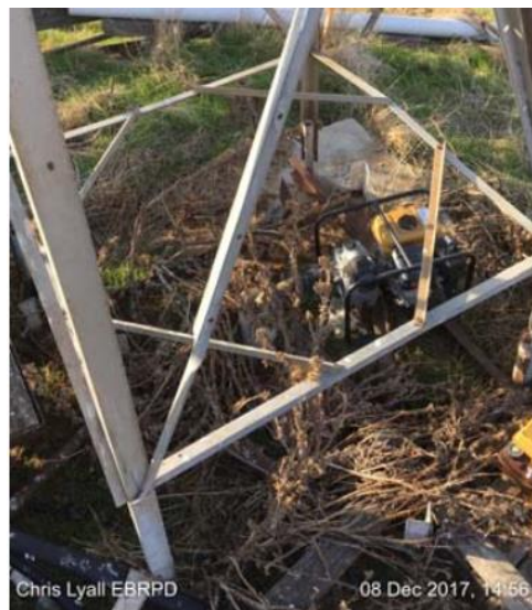
Well to be restored and debris to be removed.
