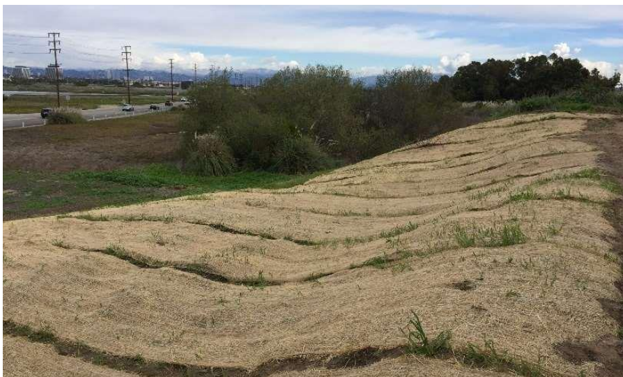
Installation of erosion control mats on hillside in restoration area
