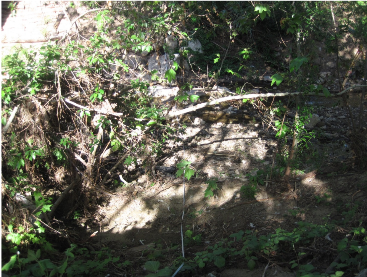
Photo C-4. San Jose Creek (Route 101, PM 21.63) tailwater control point downstream of crossing.
