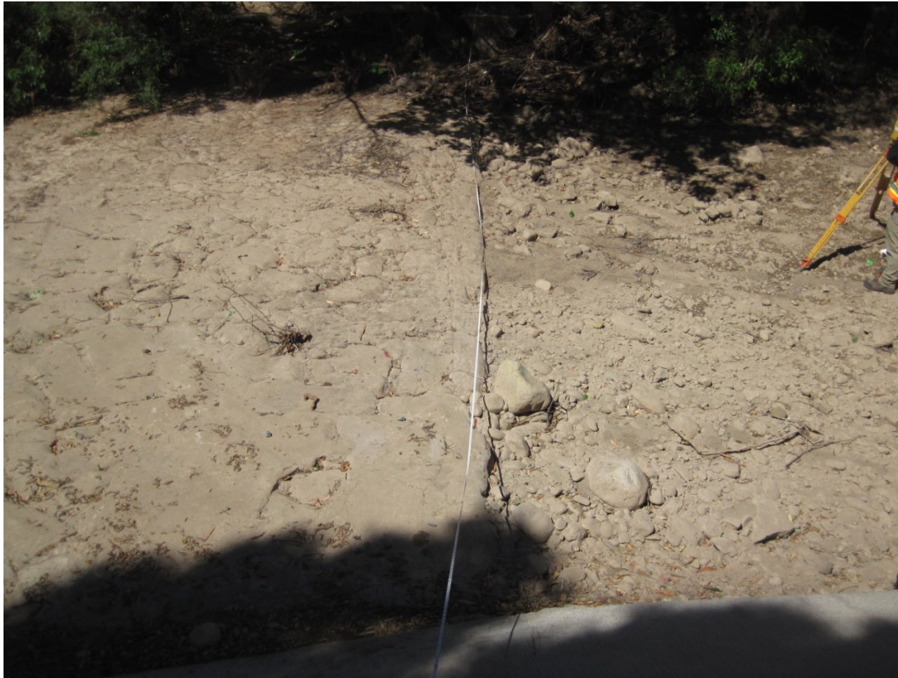
Photo C-3. Maria Ygnacio Creek (Route 101, PM 20.95) no tailwater control point; break in natural streambed channel downstream of crossing.
