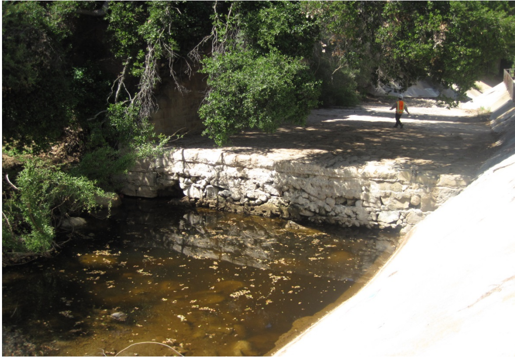
Photo 4. Route 101 (PM 20.95), looking upstream at abrupt channel elevation drop approximately 250 ft. downstream of surveyed crossing.
