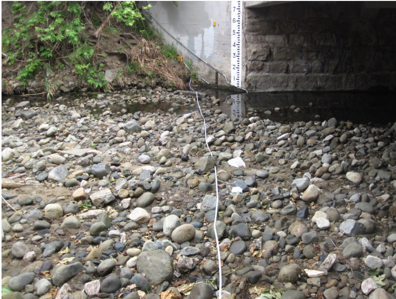
Photo C-2. Mission Creek (Route 101, PM 13.96) tailwater control.
