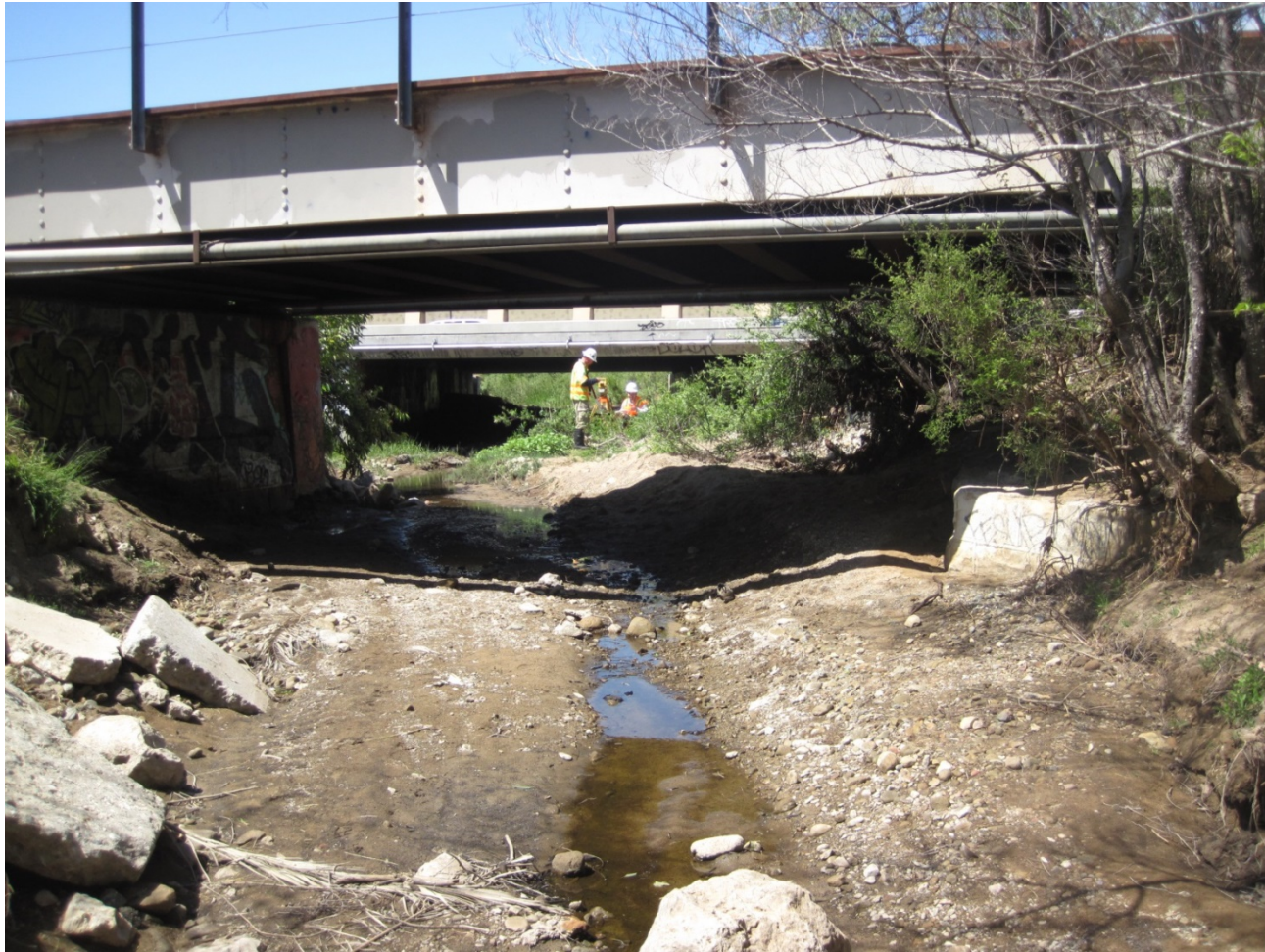
Photo C-1. Downstream looking upstream at Sycamore Creek (Route 101, PM 12.34) no identifiable tailwater control.
