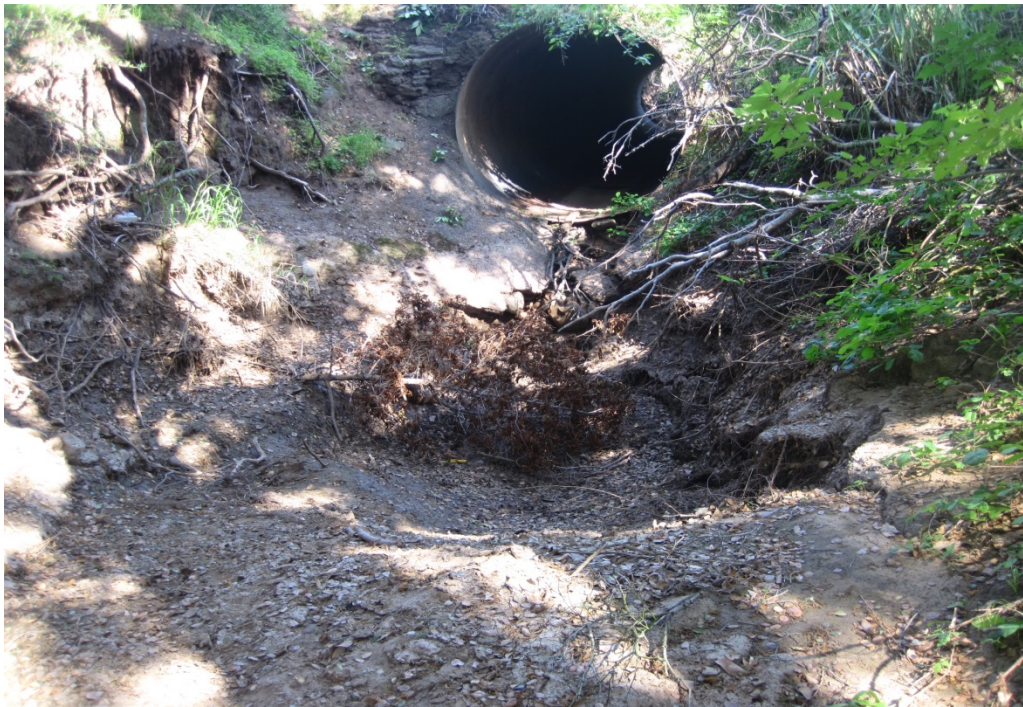
Photo 6. Route 192 (PM 0.37), Cieneguitas Creek, looking upstream at outlet drop.
