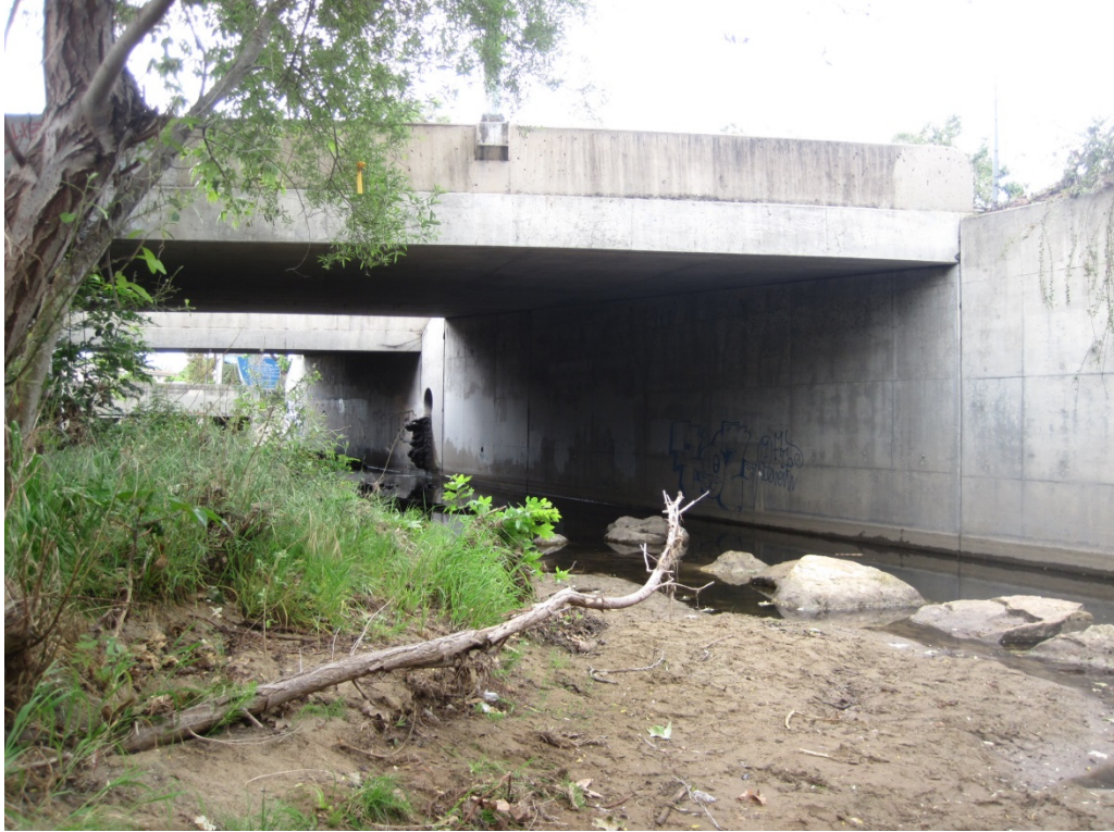
Photo 2. Route 101 (PM 13.96), looking upstream along Mission Creek.
