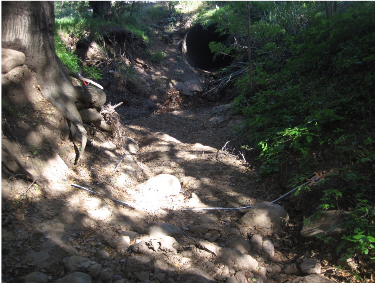
Photo C-5. Cieneguitas Creek (Route 192, PM 0.37) tailwater control point downstream looking upstream.
