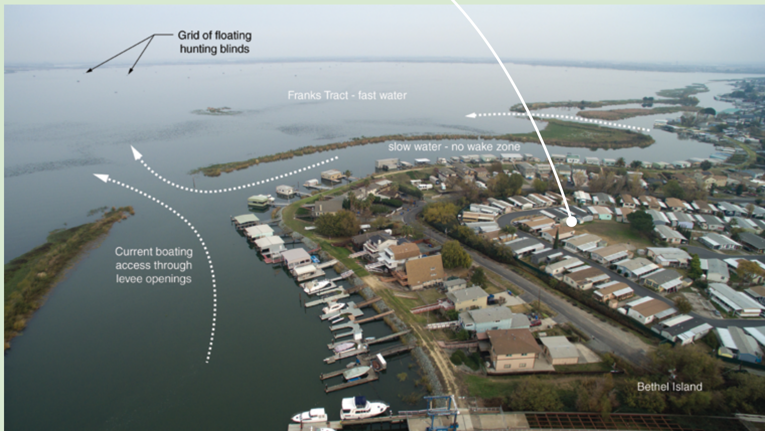
After reviewing the CDFW restoration approach, a local resident proposed a design for preserving access to existing channels, adding recreational amenities, and locating tidal marsh habitat farther away from the Bethel Island shore. This design approach received general support during a meeting with the Bethel Island community on January 5th. Local design drafted by David Gloski. Annotated aerial image Brett Milligan.
