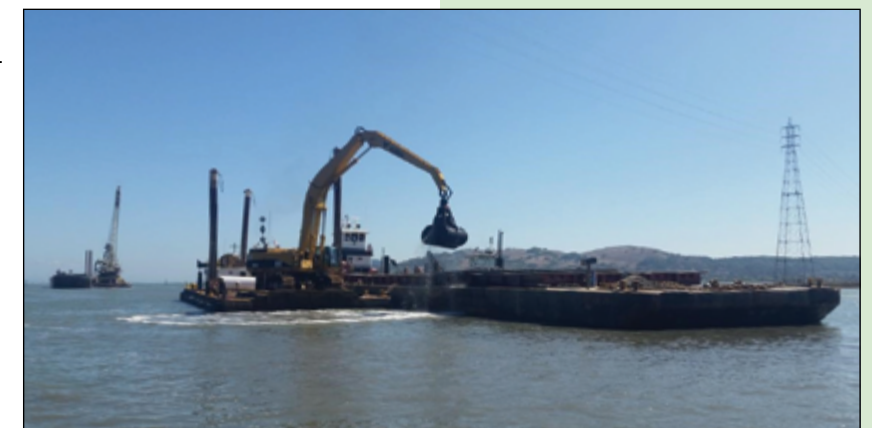
Dredging operation. Photo courtesy Moffatt & Nichol
