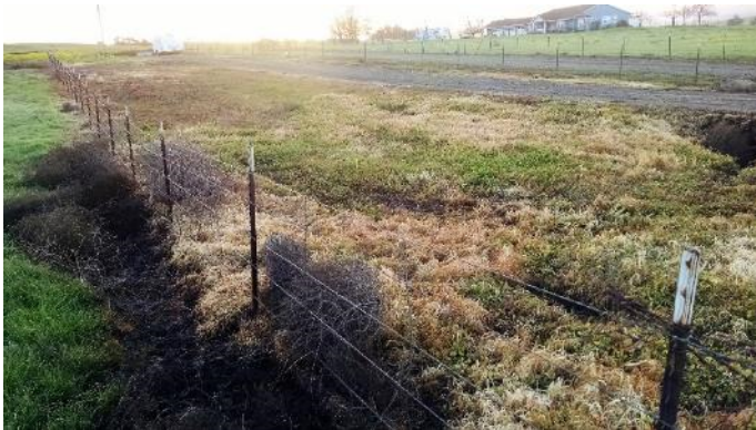
Photo 9. Fences along cattle pastures north and east of Dagnino Road within segment R700. The drainage swale passes underneath a gravel driveway leading to a private resident visible on the right side of the photo. Taken facing E. (2/19/16)
