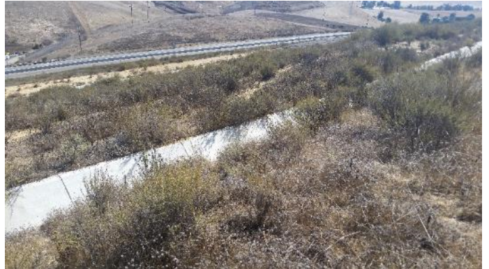
Photo 2. Concrete drainage feature at the northern end of the assessment area. (10/19/16)
