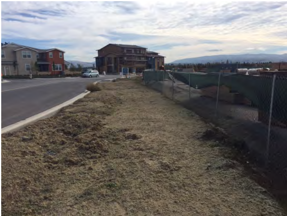
Photo 1016: View to imported fill west of access road, with paved roadway and newly built houses. Photographed by Joanne Grant on 11/7/2016.
