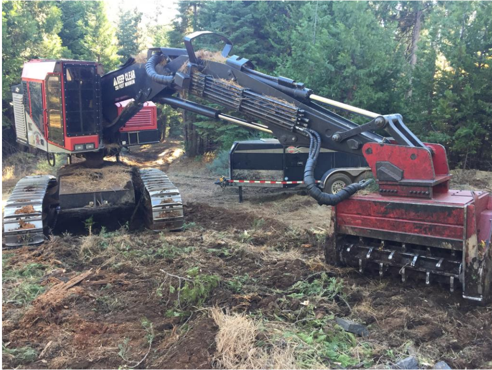
One of the masticators on the project site.
