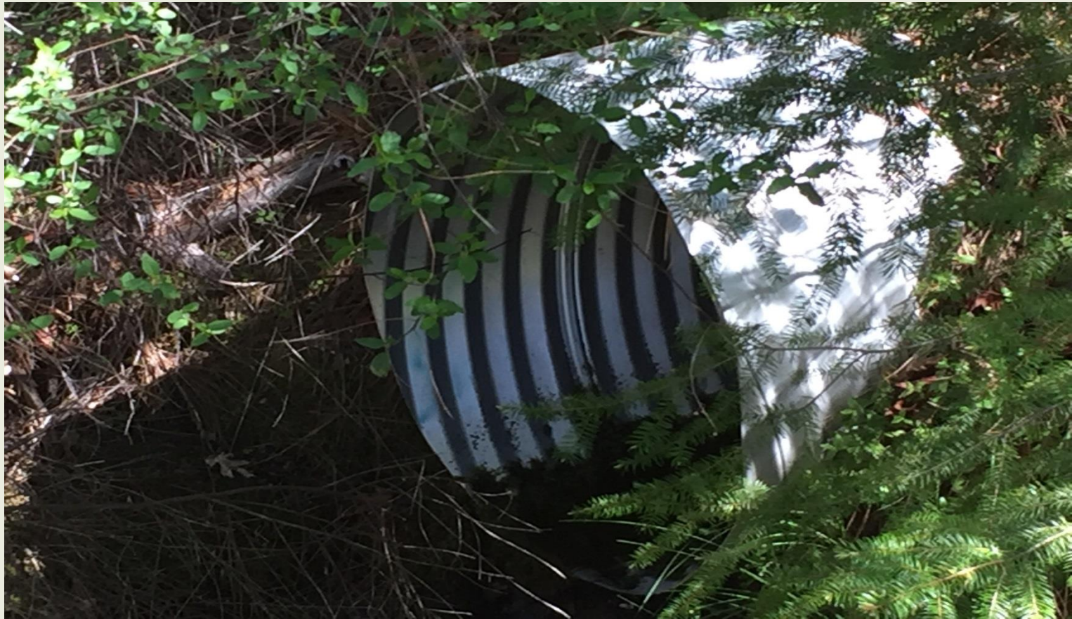
Typical aluminum culvert proposed for removal
