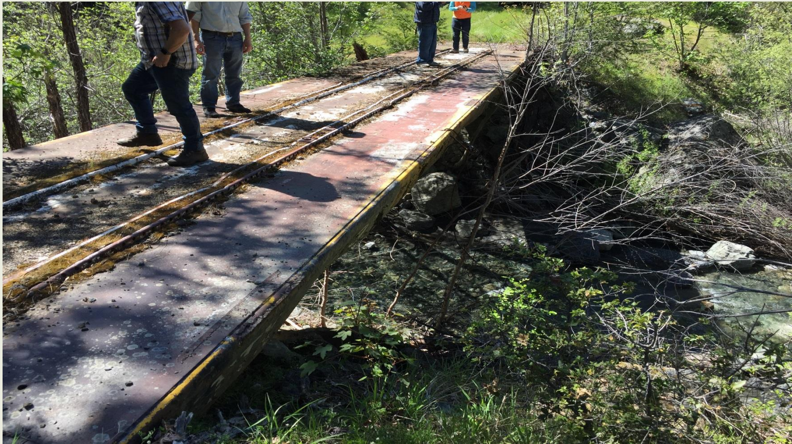
Bridge proposed for removal
