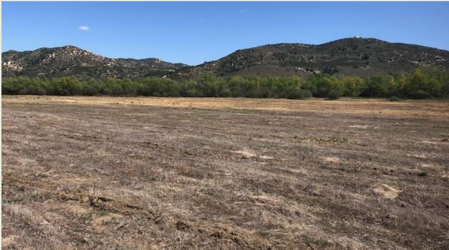
Project area after site prep
