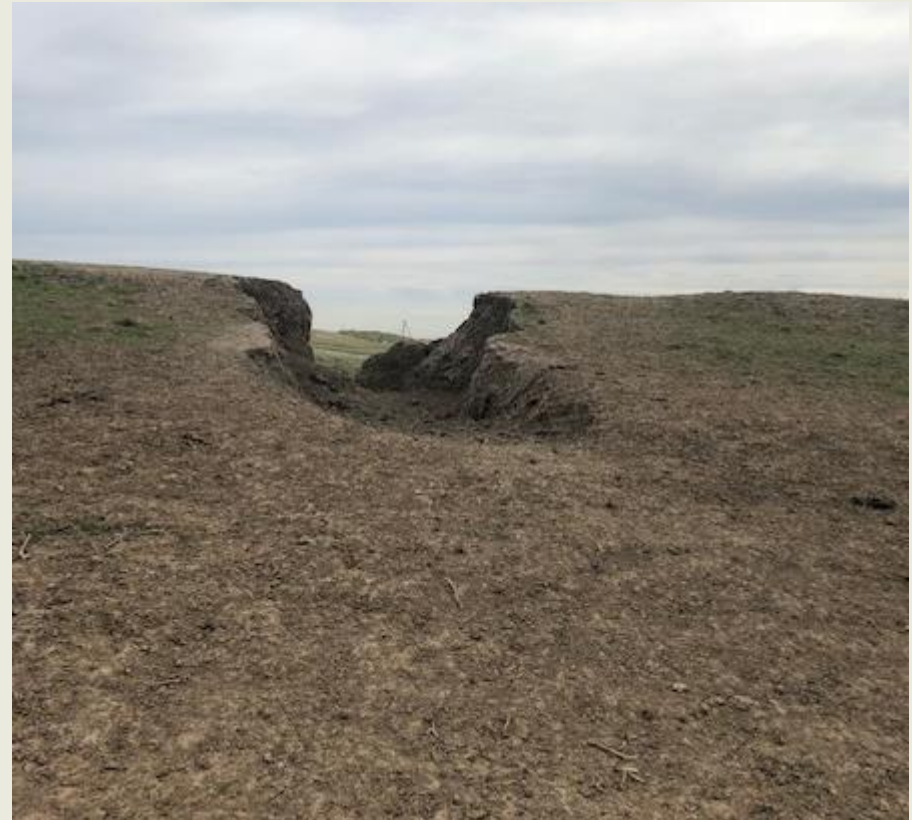
Large Stock Pond On Site With Failed Berm
