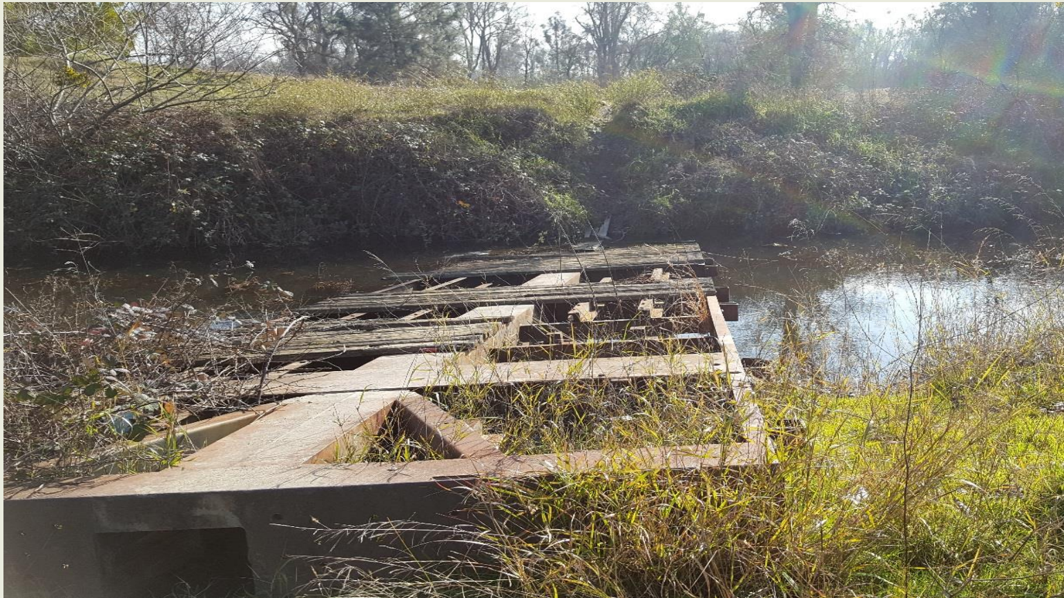
View of one of the existing interior canal crossings
