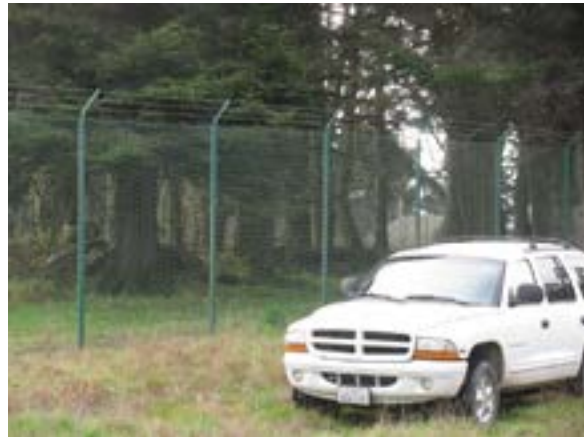
Airport Chain-Link Security Fence
