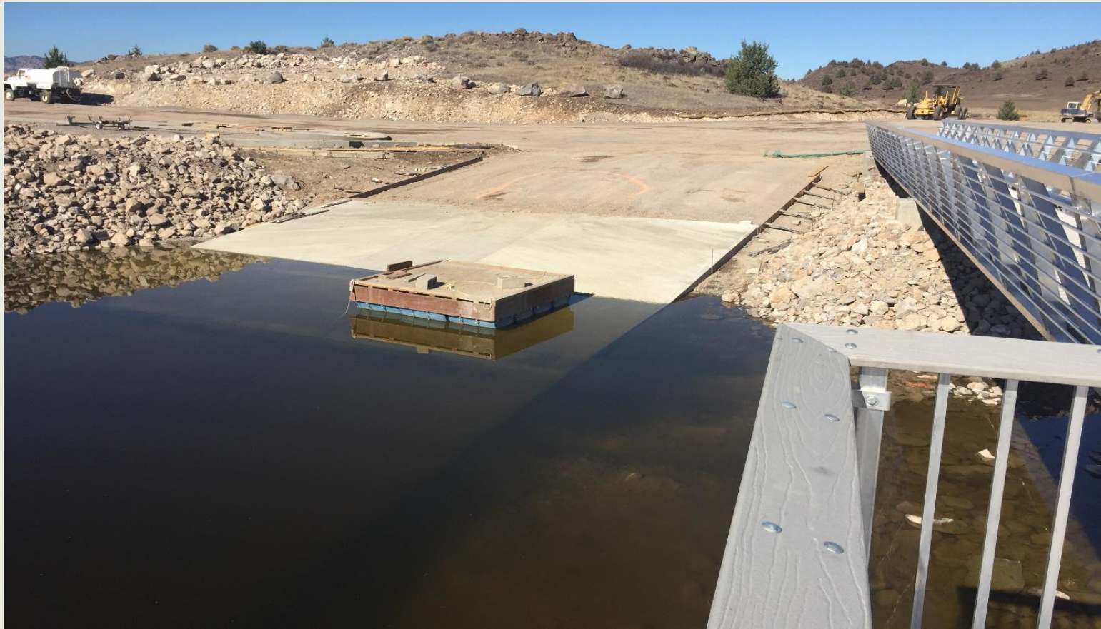
New ramp looking back from fishing pier.
