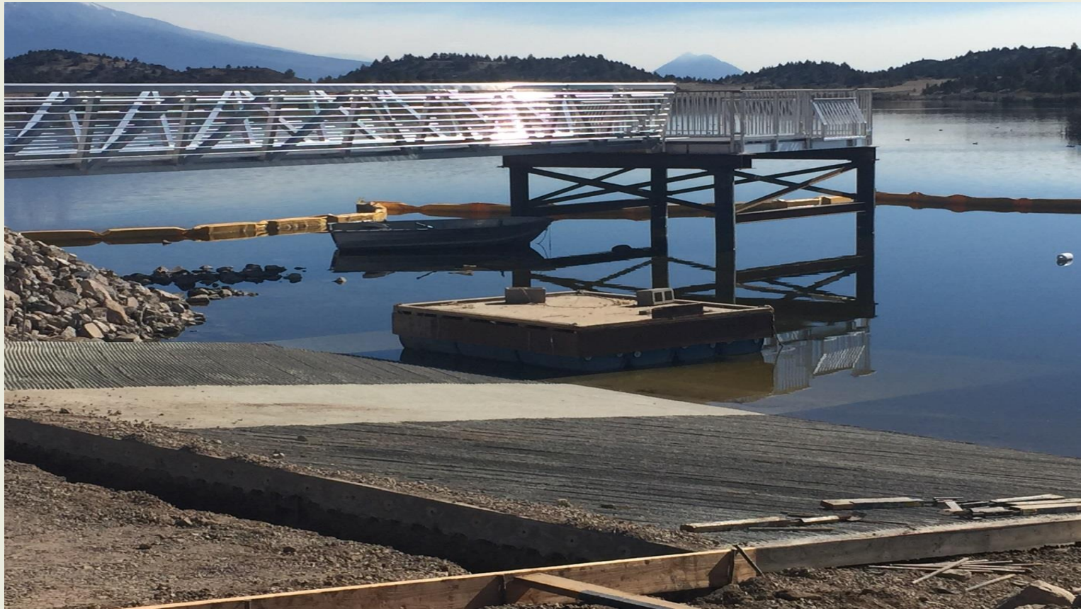
New ramp and fishing pier.
