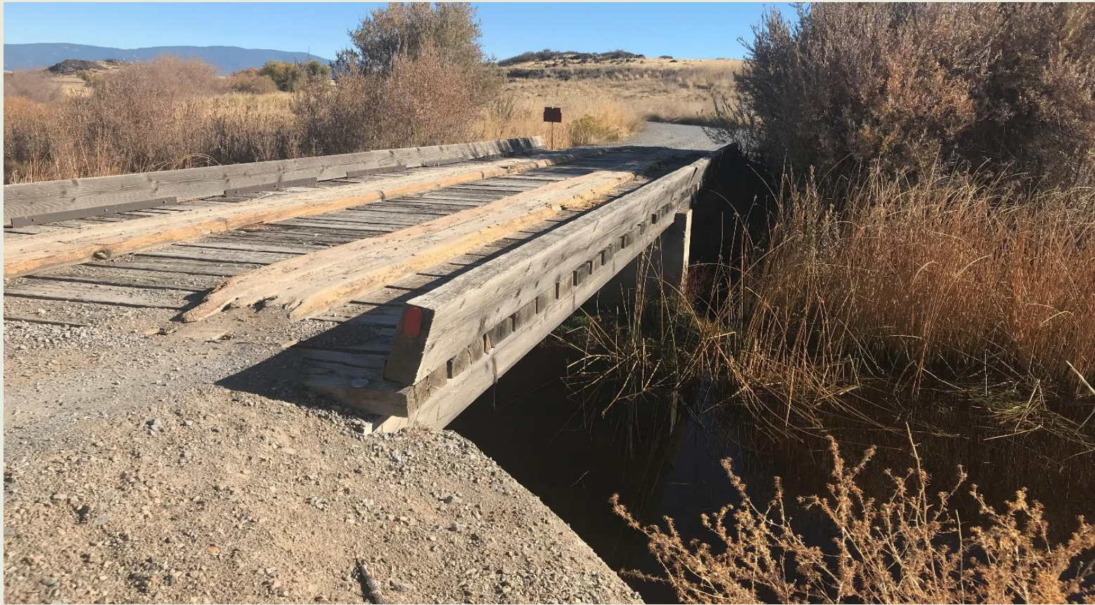
Existing bridge looking south.
