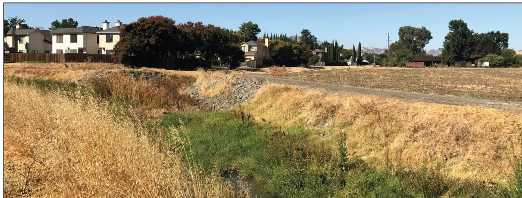
Three Creeks Parkway Project at the confluence of Sand and Marsh Creeks. Photo courtesy Contra Costa County Flood Control and Water Conservation District
