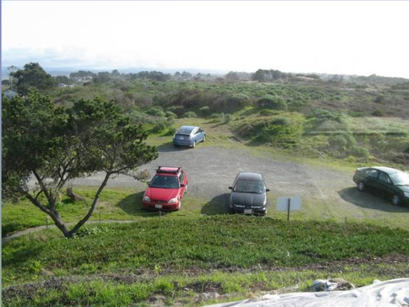
View from cupola on top of Nature Center overlooking where restrooms will be added (lower portion of picture) and where parking lot improvements will be made for staff.
