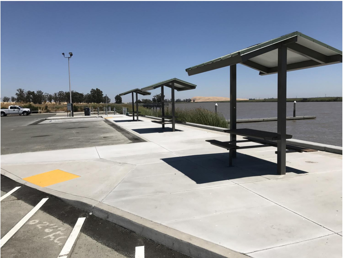
Figure 1: ADA Compliant table structure, stop curb, and accessible parking stall interface after construction. Image also contains light pole and interpretive kiosk in distance.
